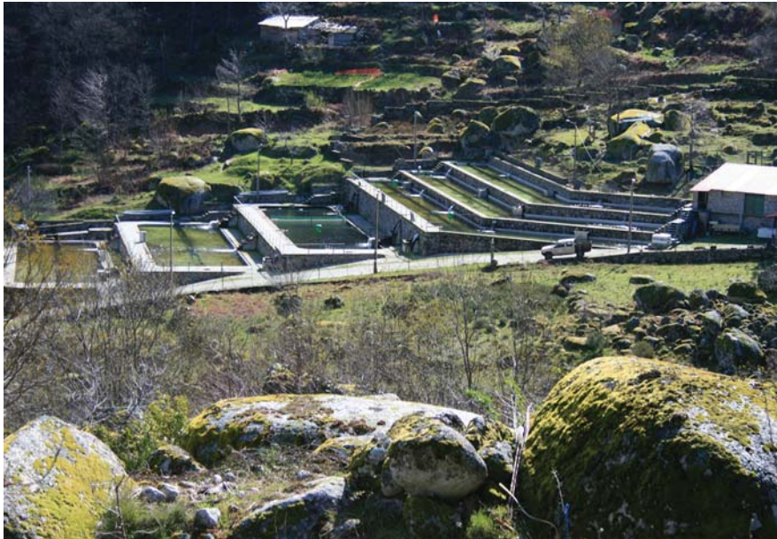
Figure 5.20: The Existing Water Pools, View from the West.
