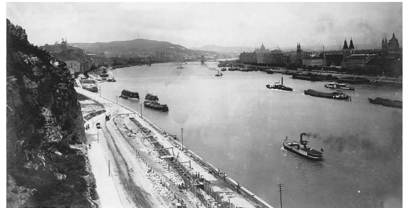
Fig. 4.27. The Construction of the embankment near Gellért Hill.
