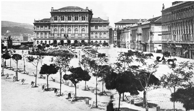
Fig. 5.16. The square after the coronation ceremony with the mound at its centre and two new rows of trees. The Academy of Sciences can be seen in the background.
