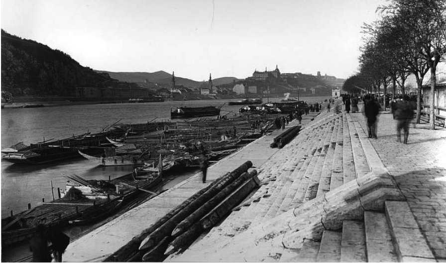
Fig. 4.2 (left) The Franz Joseph embankment in Pest shows lumber unloaded for further transportation (1894).
