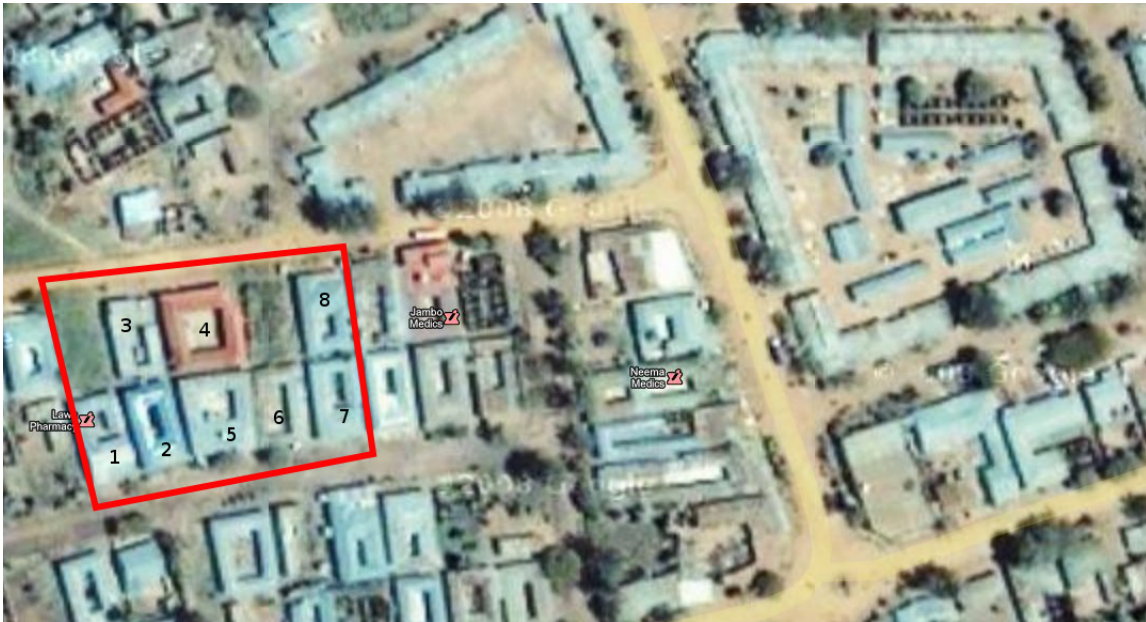
Figure 4.4: Aerial view of the town of Mugumu, Tanzania for context. The main intersection is in the lower right while the large quadrilateral group of buildings in the upper right is the town market. The buildings used for the simulation are highlighted and numbered on the left side of the image. ©2012 GeoEye, Cnes/Spot, Digital Globe, & Google
