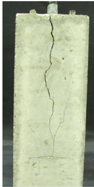
b) Post-failure cracking
