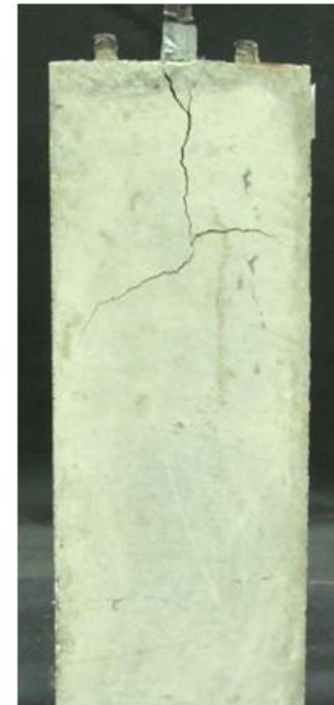
b) Post-failure cracking
