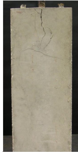
b) Post-failure cracking
