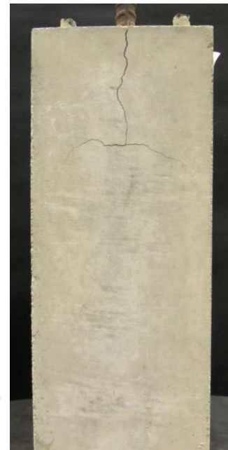
b) Post-failure cracking
