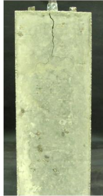
b) Post-failure cracking
