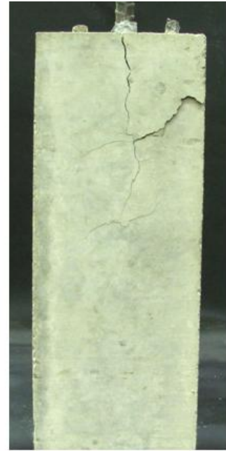
b) Post-failure cracking
