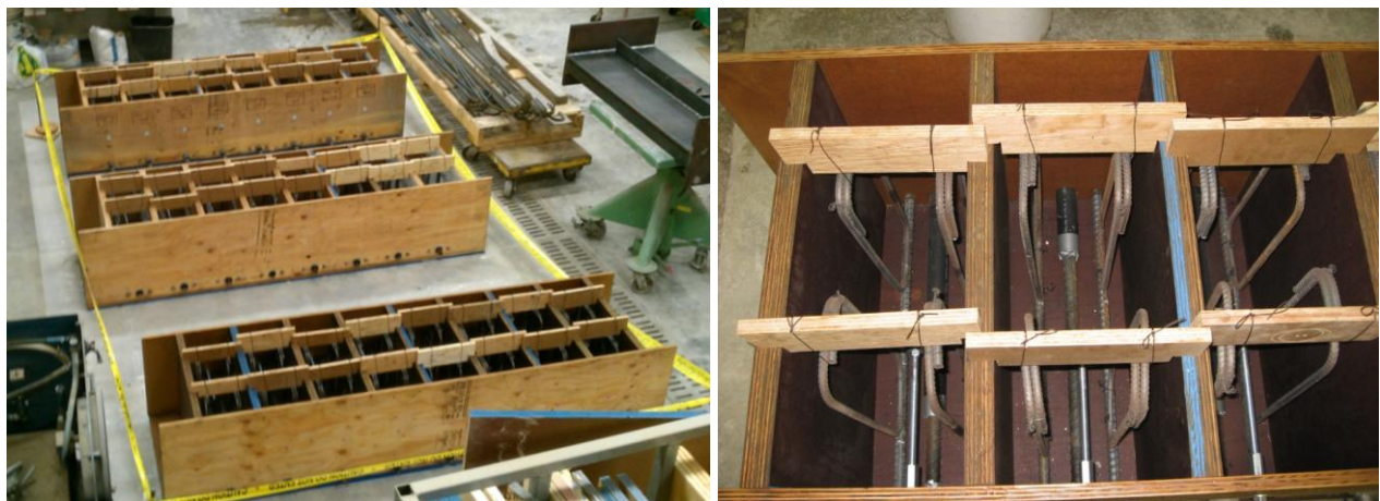
Figure 9.5 Typical beam-end formwork casting beds and reinforcement
