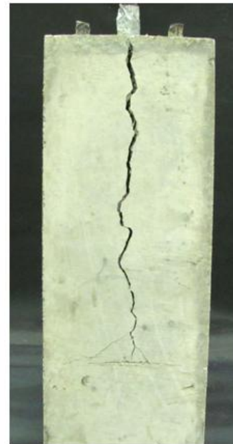
b) Post-failure cracking
