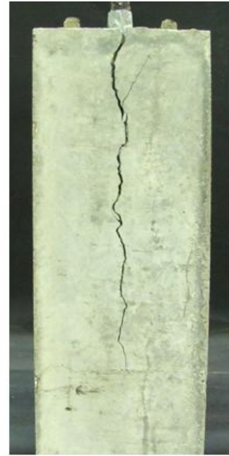
b) Post-failure cracking
