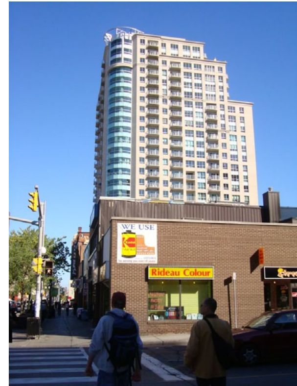
FIG. 3.7 CLARIDGE PLAZA One of the larger recent condominiums in Ottawa, along Rideau street.
