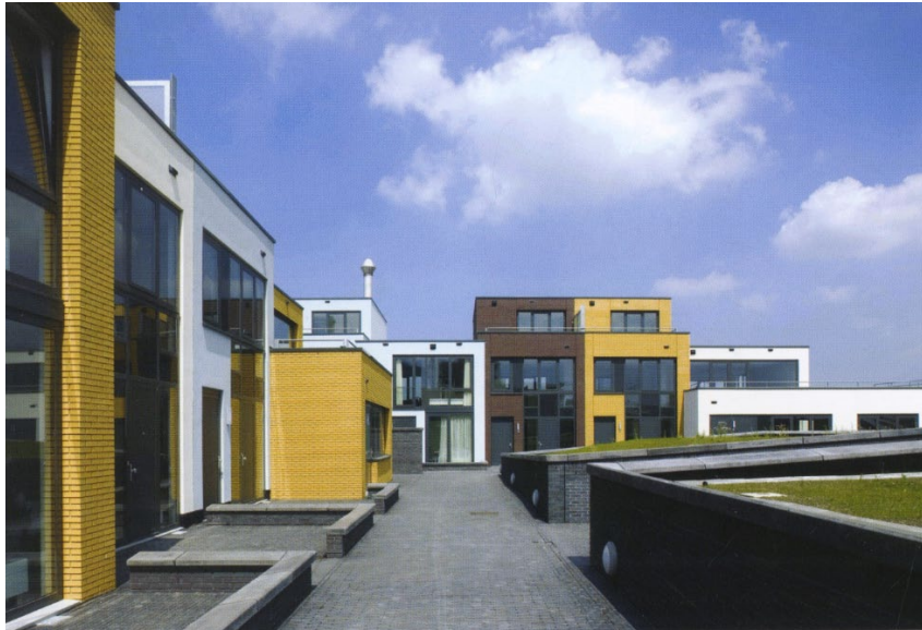
FIG. 4.51 ROWHOUSES AT ROOF LEVEL
