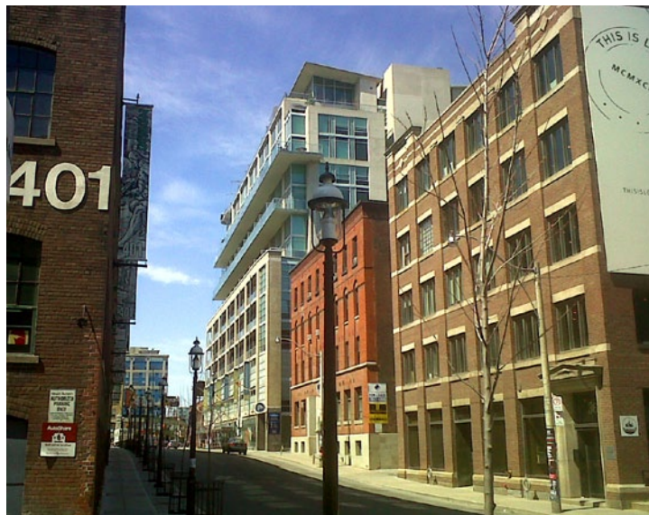
FIG. 4.82 DISTRICT LOFTS FROM RICHMOND ST.
