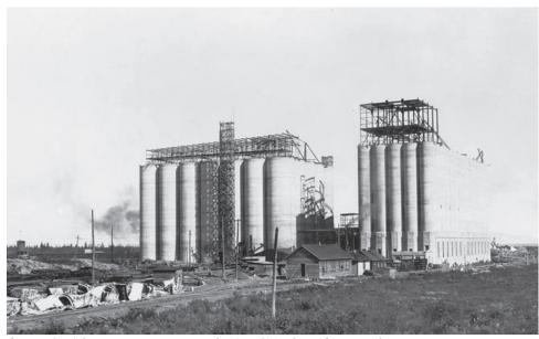
figure 1.49 \_ The concrete construction the Grand Trunk Pacific terminal grain elevator was the first of its kind in Fort William
