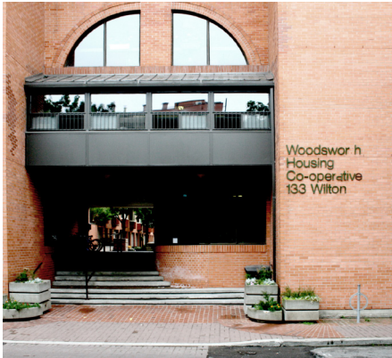
figure 4.12 Woodsworth Housing Co-operative
