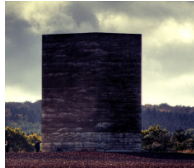
figure 3.09 Rammed Concrete Exterior
