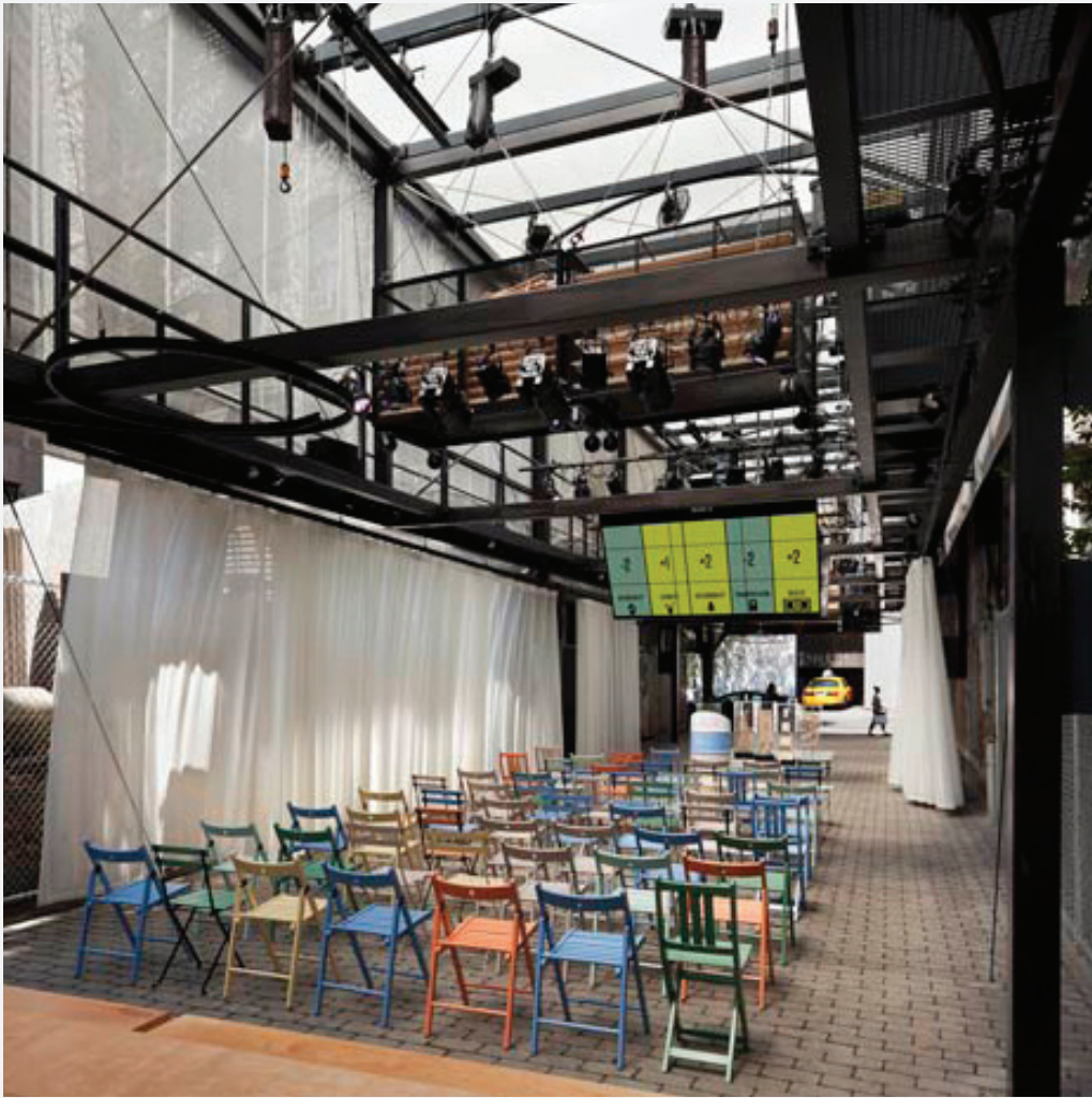
FIG 64 In this view of Atelier Bow Wow's 2011 design for BMW Guggenheim Lab, colourful wooden chairs are arranged for a discussion, beneath the fiber-glass structure that holds lights, screens, and curtains.
