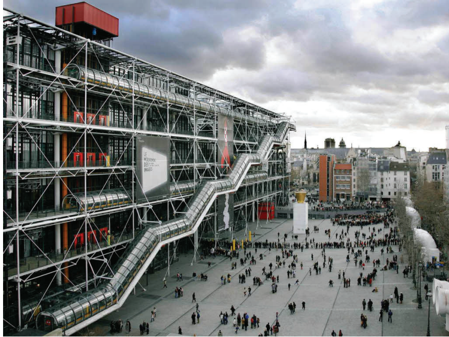
FIG 23 The Fun Palace influenced the aesthetic of the Pompidou Centre in Paris.
