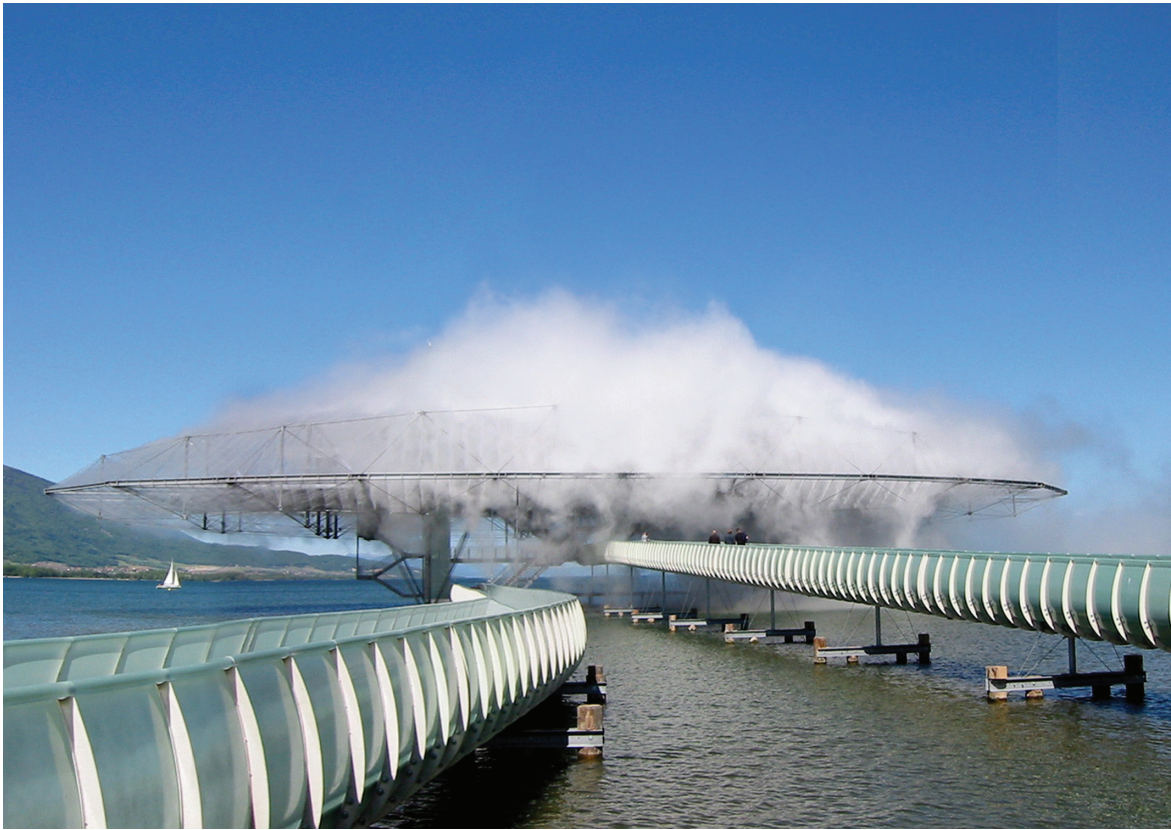
FIG 38 Above and Background: Blur is an anti-monument. The structure is but a mere shell that generate an atmosphere of mist that is controlled by computers.
