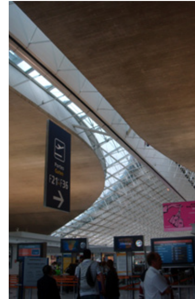
[3.48] A view of Andreu's fully-glazed triangular structure overtop the gates concourse.
