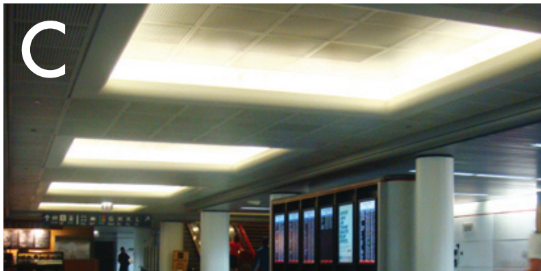
[2.91] Ambient cove lighting over the circulation spine of the gates concourse at Chicago O'Hare Airport T2.
