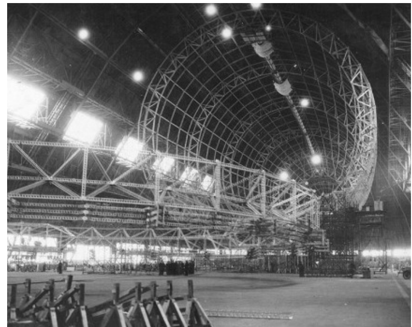
[1.1.20] The USS Macon Airship under construction at the Akron, Ohio airship hangar, c. 1932.
