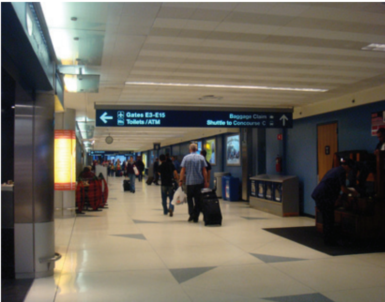
[3.1.42] A section of the gates concourse showing a low ceiling and outdated finishes.
