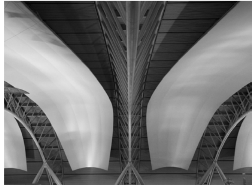
[1.1.19] A view of the roof structure over the check-in hall at Kansai International Airport. The airfoil-shaped roof promotes air circulation throughout the space.
