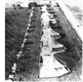
[1.1.23] An image of WWI temporary airplane hangars. The military hangar was the first building type to use tensile materials at airfields and airports.
