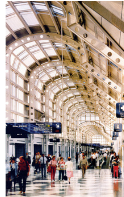
[1.1.12] The main terminal building at Chicago O'Hare's T1 bears a striking resemblance to Paxton's arcade.
