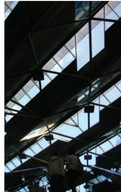
[3.79] Skylights and metal panels clad the ceiling.
