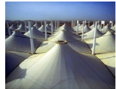
[1.1.24] King Abdul Aziz International Airport, Hajj Terminal ~ Skidmore, Owings & Merrill (1981)
