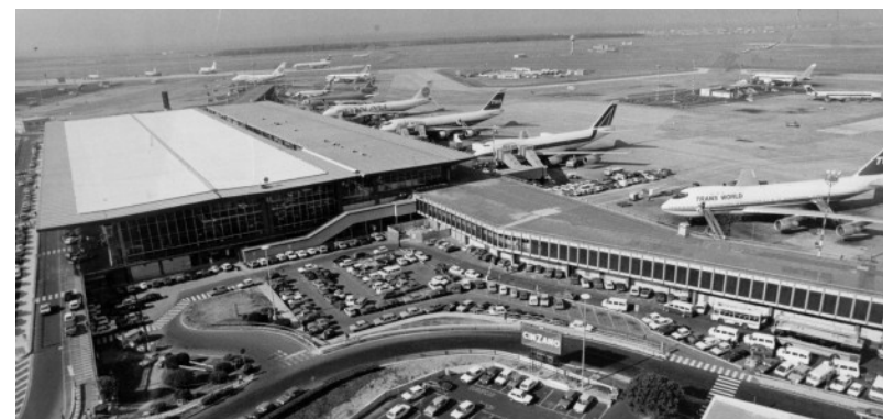
[1.66] A postcard depiction of one of the curvilinear terminals at Dallas/Forth Worth International Airport, 1970.
