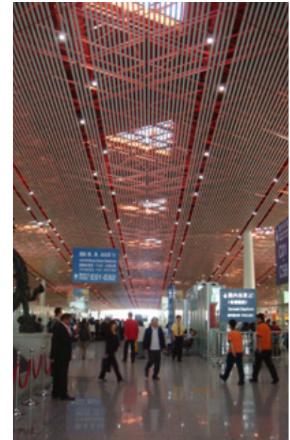
[3.98] Operable triangular skylights allow in natural light and improve air circulation.
