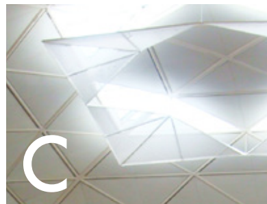
[2.80] Detail of louvre system used at MAD T4.
