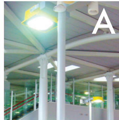
[2.90] Spotlights in the concrete roof slab at Dulles.
