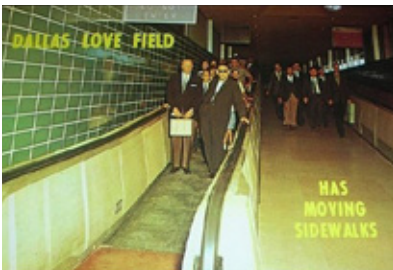
[1.57] The first moving sidewalk, or travellator, at Dallas Love Field Airport is installed in response to increased walking distances to gates, 1958.
