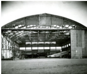
[1.1.47] An airplane hangar at Le Bourget Airfield, c. 1974. The 'elegant shed' motif is referenced in Beijing Capital's Terminal 3 and its Transportation Centre.
