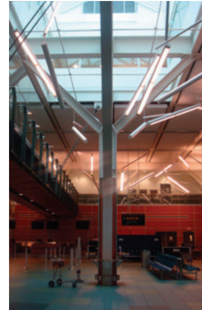
[3.1.17] Fluorescent tubes have been attached to structural trees, displaying the design's playful side.
