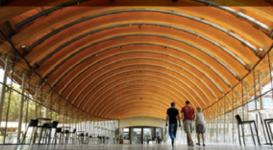
[4.80] Crystal Bridges Museum of American Art ~ Safdie (2011) Curved glulam beams provide roof support, as well as a natural feel.
