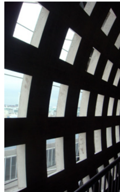
[3.49] A similar concrete aesthetic used to exist at its sister terminal, T2E, before collapsing due to weight.
