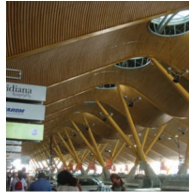
[3.39] Circular skylights allow in direct sunlight.
