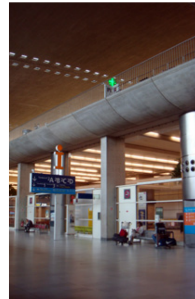
[3.50] The terminal, as viewed from the lower level. It was surprisingly empty considering its enormous size.
