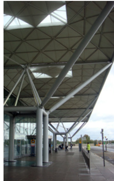
[3.69] The extension of the modular roof system over the curb provides cover from the elements.
