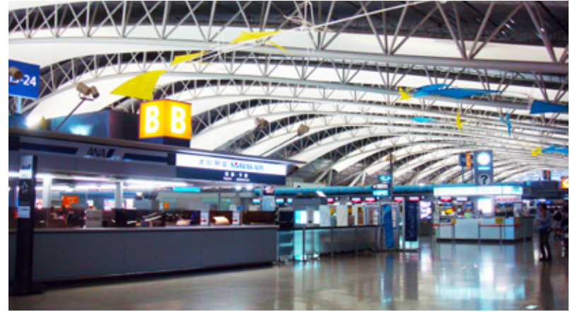
[3.1.6] Kansai Airport's check-in hall is shaped like an airfoil to promote good air circulation.
