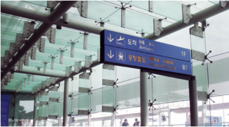
[3.1.2] Structural glazing is used to cover a series of escalators between the arrivals and departures levels.
