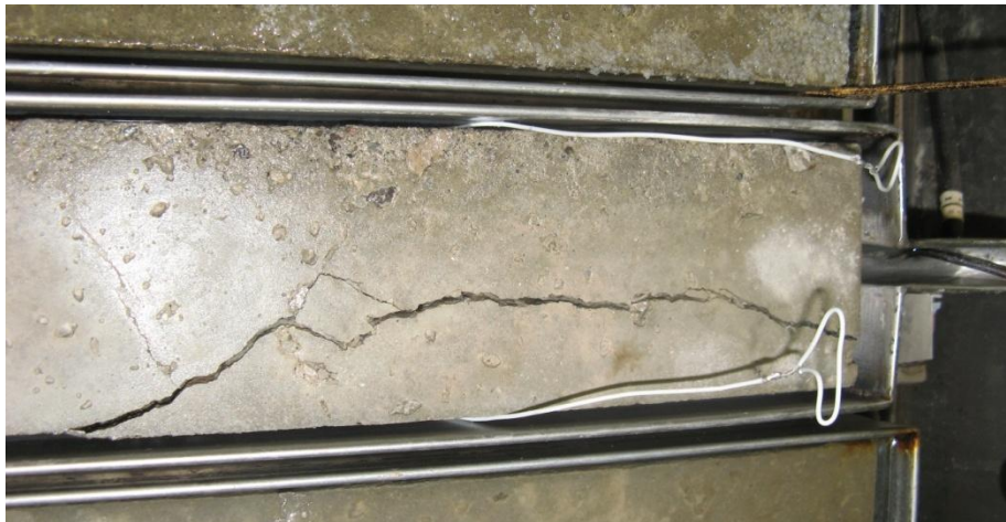
Figure 5.1-6 - Severe crack in freezing and thawing Set 1 temperature control prism
