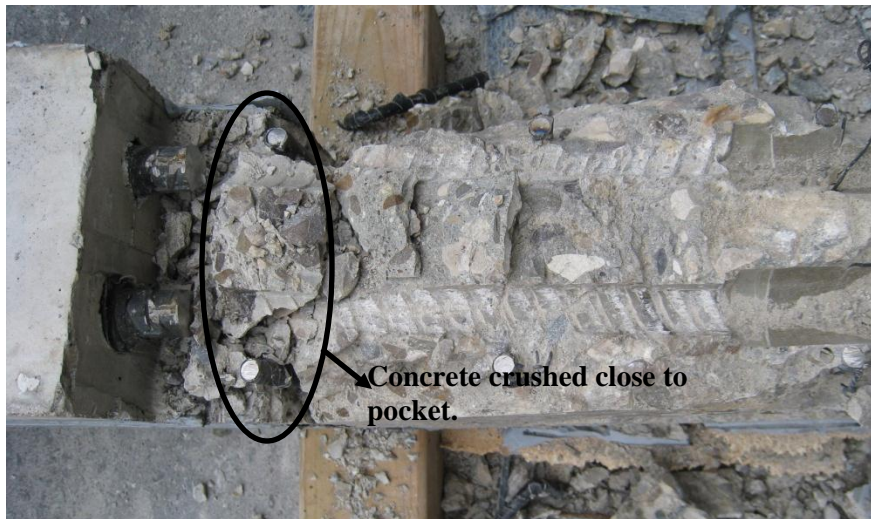
Figure 5.9: Beam M-200-R-n after failure and removing the bar from the anchorage zone. The beam was turned upside-down.
