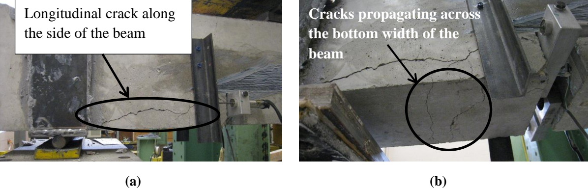
Figure 5.28 Cracks in the bonded length of Bream M-350-U-n along (a) side of the beam and (b) bottom of the beam.
