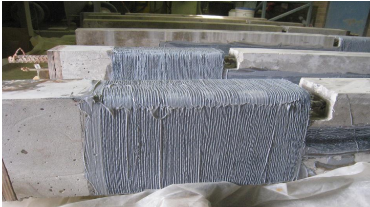
Figure 3.11 A repaired beam turned upside-down.
