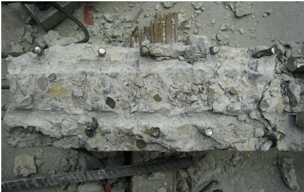
Figure 4.27 Concrete keys crushed along the anchorage zone for Beam M-B-100-0-2. This beam is turned upside-down.
