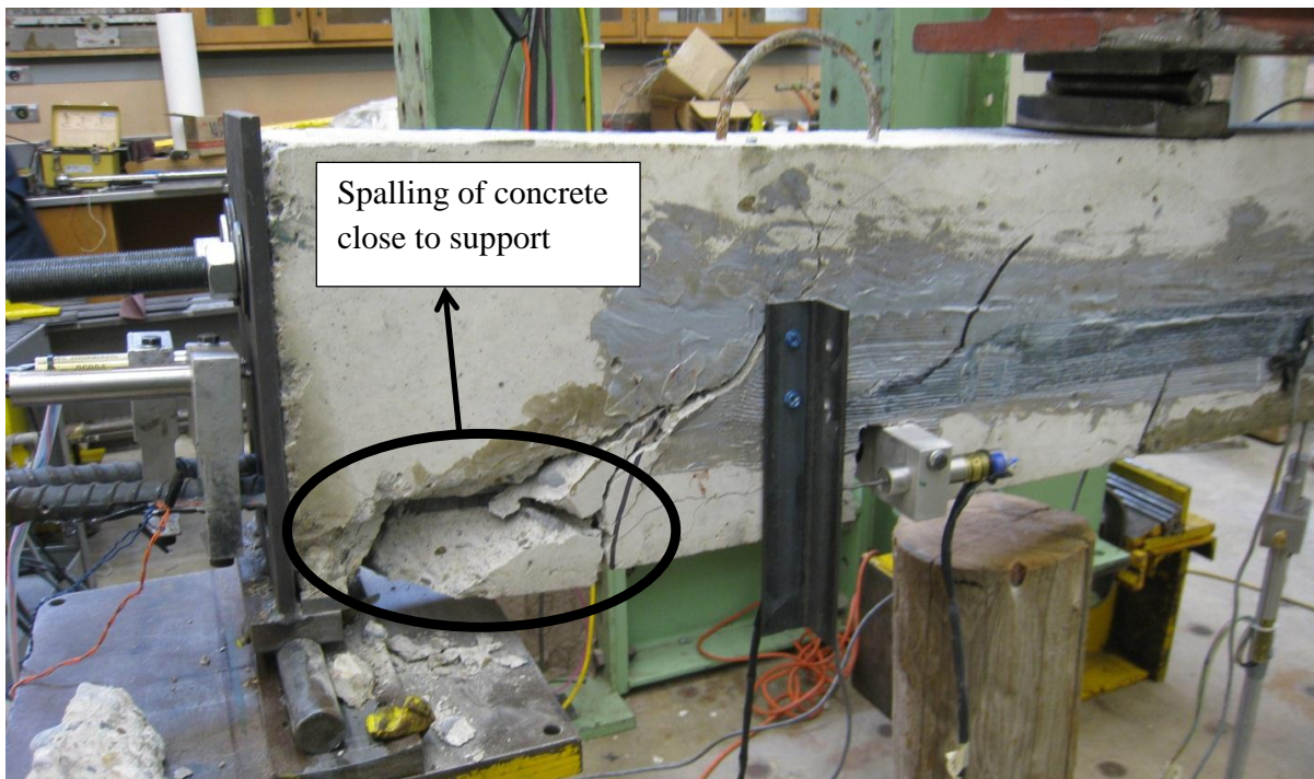
Figure 4.34 Beam F-A-64-0 close to failure in the testing frame showing the concrete close to the support spalling.
