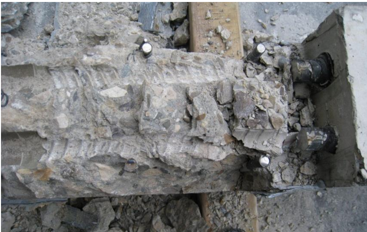
Figure 5.21 Beam M-200-R-n after failure and removing the reinforcing bars to the concrete keys. The beam was turned upside down.
