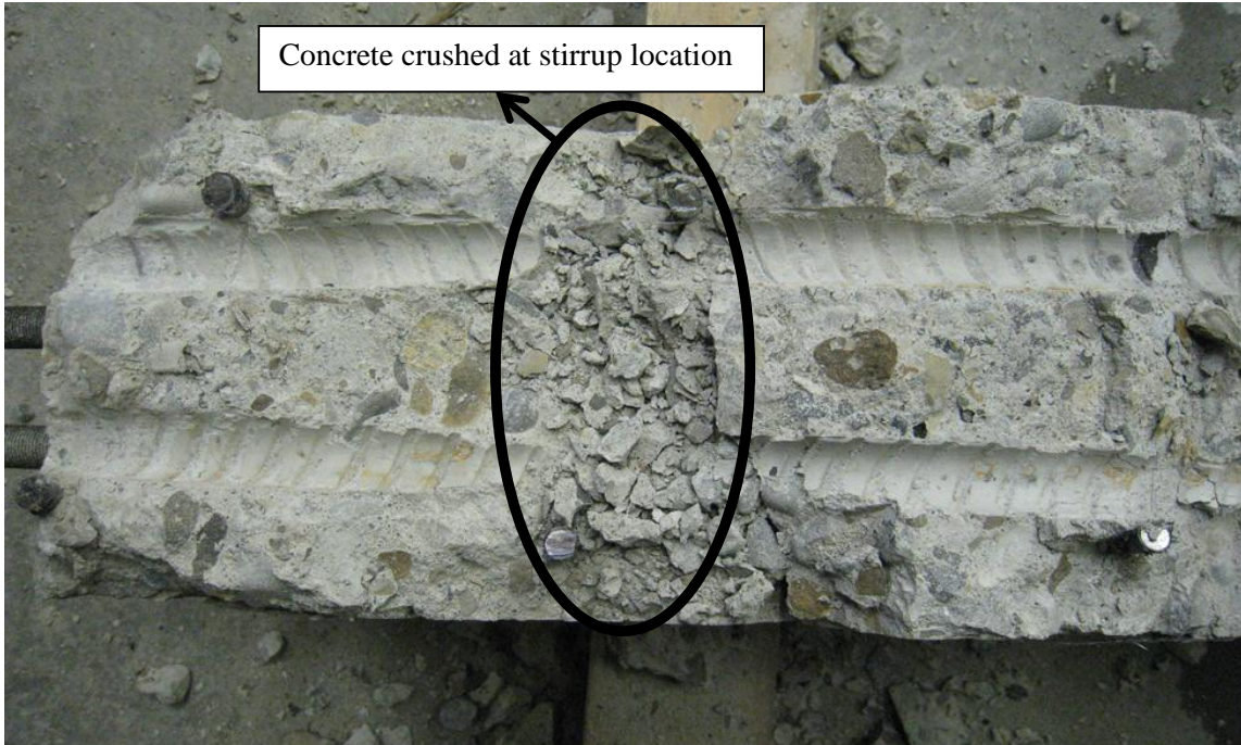
Figure 4.35 Beam F-A-64-0 after failure and removing the reinforcing bars. The beam was turned upside-down.
