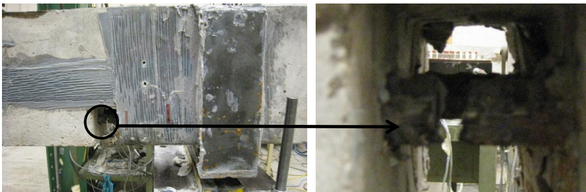
Figure 5.48 Beam F-200-R-m-72 failed by bar rupture in the pocket.
