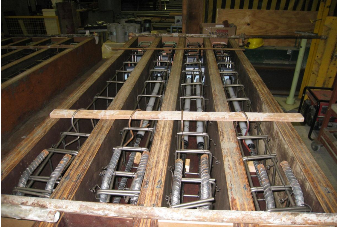
Figure 3.9 General view of the cages in the formwork before casting.
