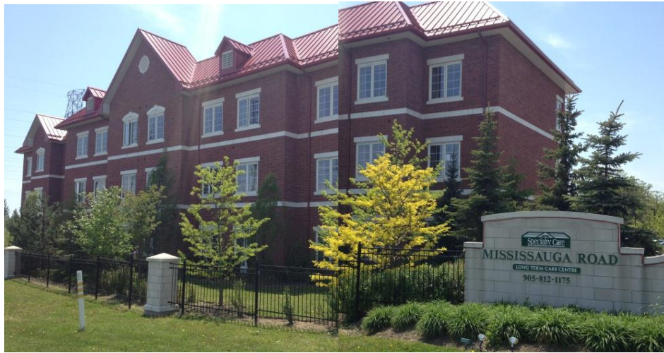
Images 6 and 7: Mississauga road LTC home exterior side (top); Exterior front (bottom)
