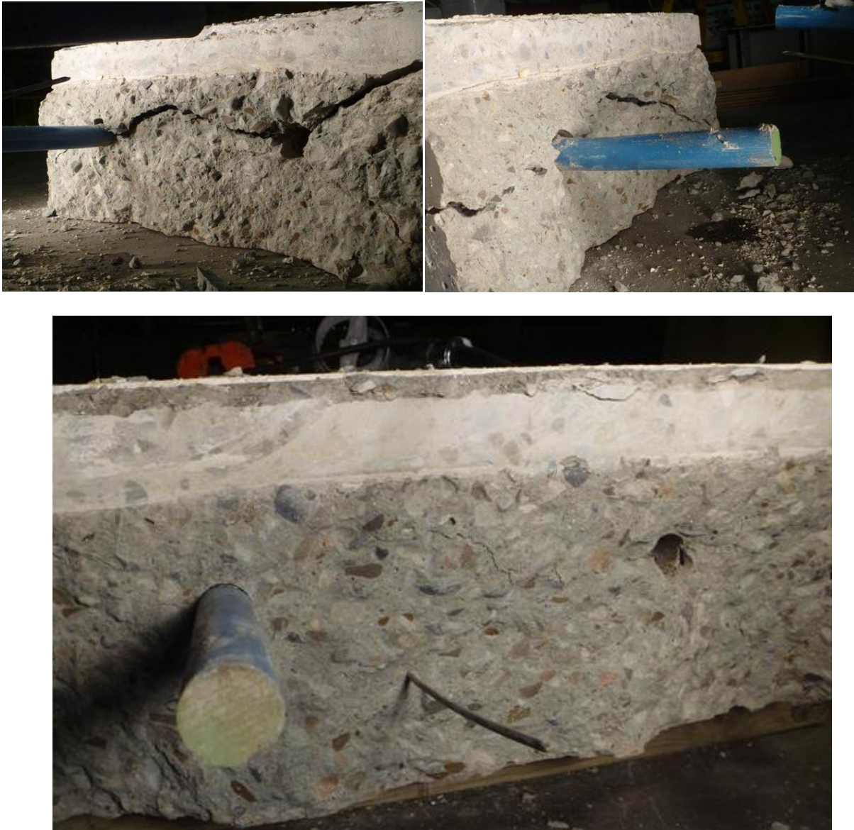
Figure 6-23 – Dowel Bar Specimen: Slab Joint Face Showing Damage Extending from Dowels
