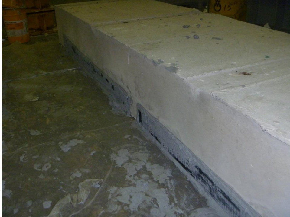
Figure 6-15 – Sika S512 Carbodur Strips attached
