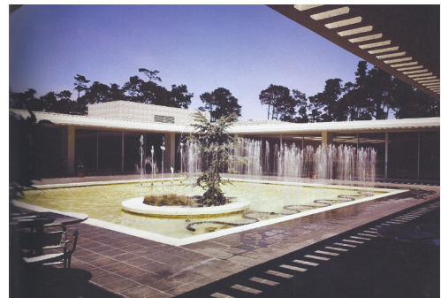
Fig. 60 Community Hospital of the Monterey Peninsula Courtyard
