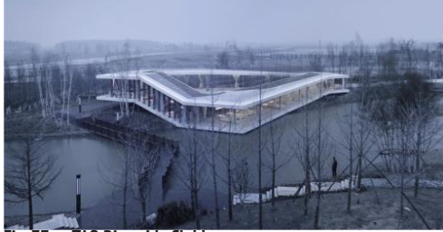
Fig. 77 TAO Riverside Clubhouse
