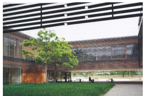
Figs. 61 REHAB Basel Entrance Courtyard, Herzog and De Meuron
