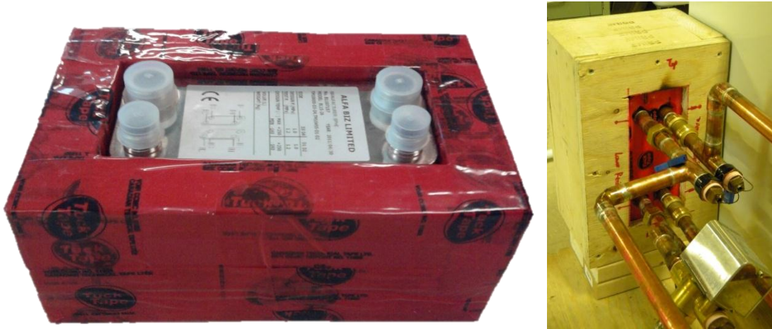
Figure 3.12 Heat exchanger with insulation (left) and installation (right)
