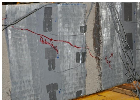
Figure 5-36: Diagonal tension shear crack propagation of beam 430G-300-NA
