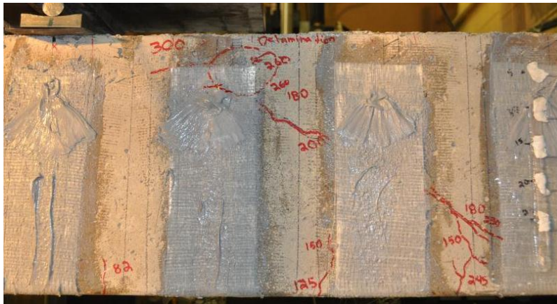
Figure A-20: Crack propagation around FRP anchor
