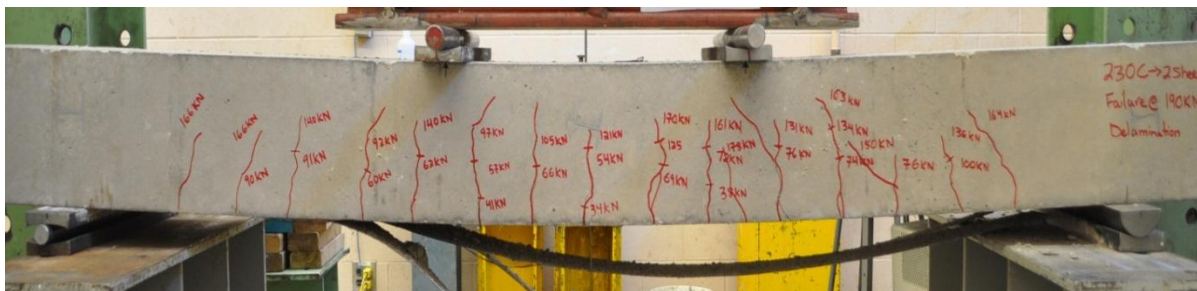
Figure 6-1: Flexural failure of slab 230C-2L-NA
