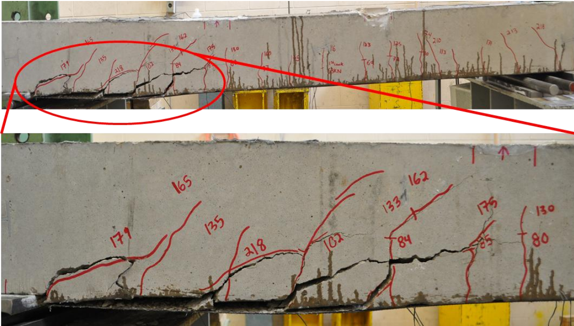
Figure 6-6: Failure of slab 600C-2L-8A
