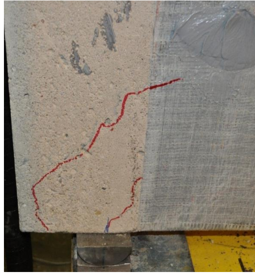
Figure 4-27: Diagonal tension end anchorage failure of beam PC-430G-800-A
