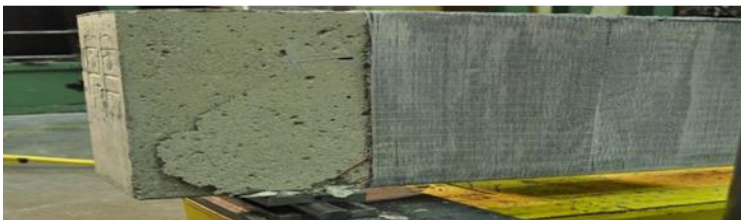
(f) – Diagonal tension end anchorage failure
