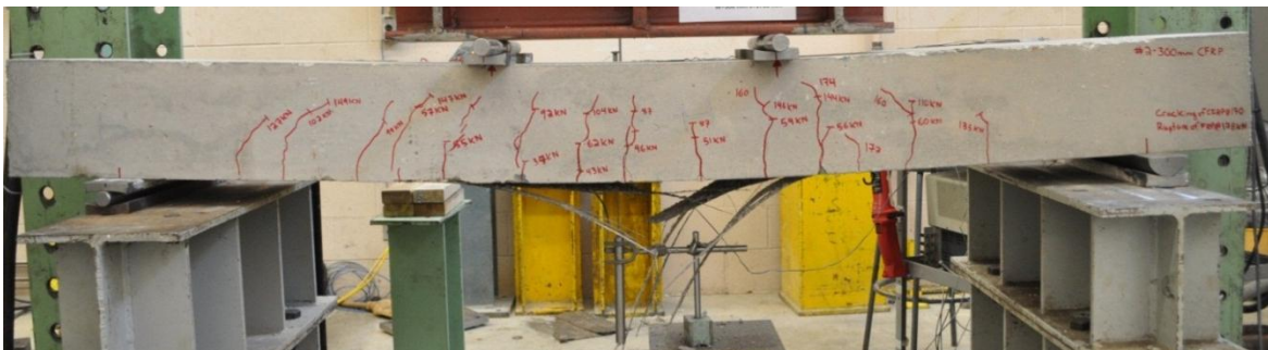
Figure 4-44: FRP rupture of 230C-1L-NA
