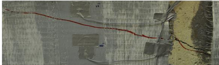
(b) – Loss of aggregate interlock
