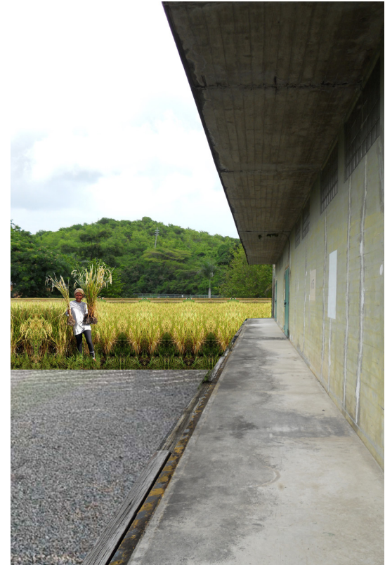
Fig. 185 Agricultural Landscape surrounds the hostel bunkers.
