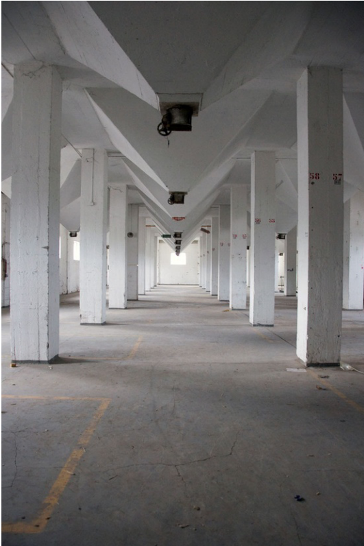
Fig. 186 Inside the rice silo bunker.
