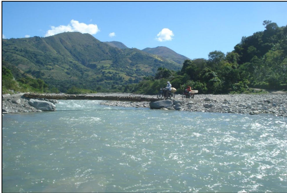
Figure 21: An artisanal bridge constructed of logs, the first of the four river crossings needed to reach El Recodo
