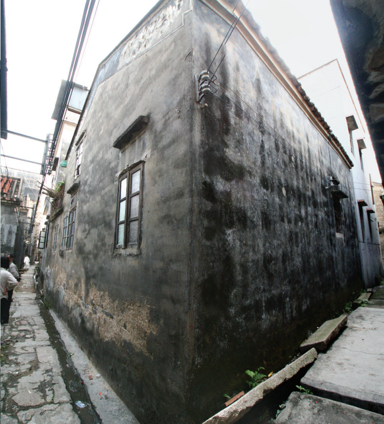
Note the cement rendering of the two homes are covered over together as if a single structure.
