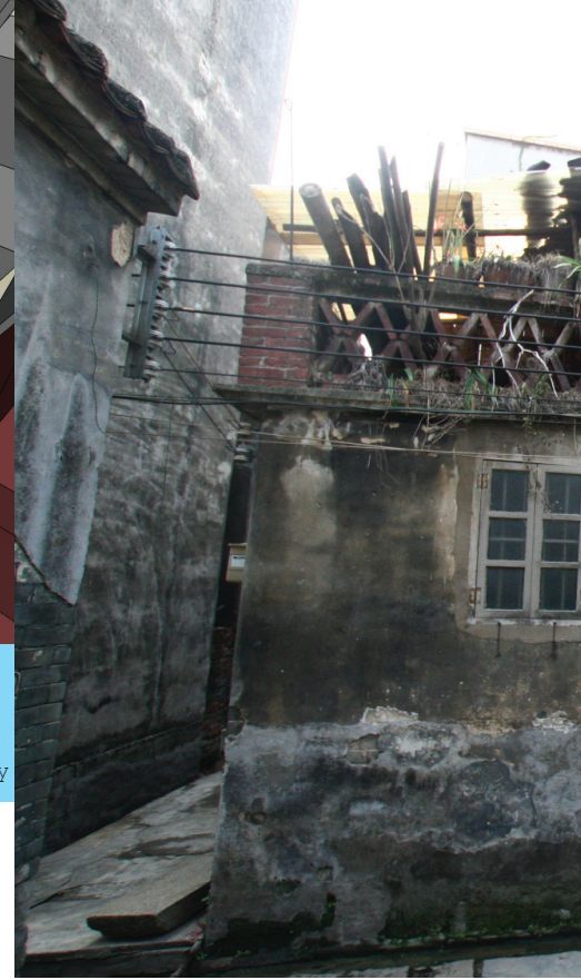
Fig. 282. Typical brick village house. Photograph.
