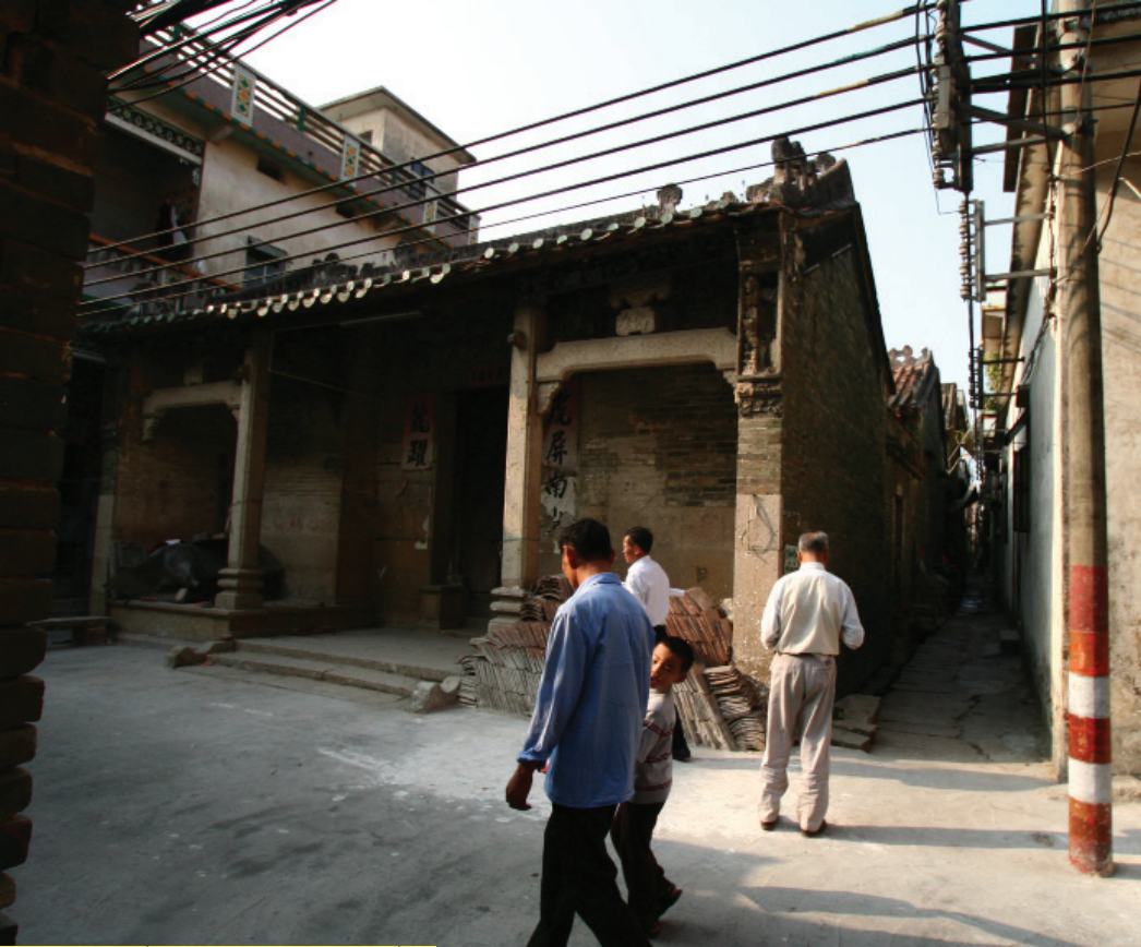
Clan shrines along the arterial streets serve as public spaces for congregating.
