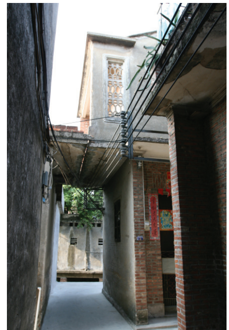
Fig. 305. Another example of terrace over laneway.
