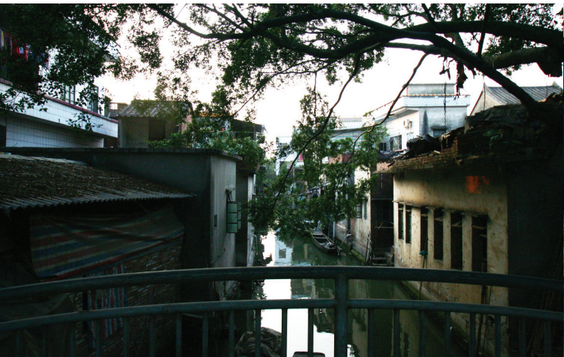
Fig. 352. Canal X before. Photograph.
