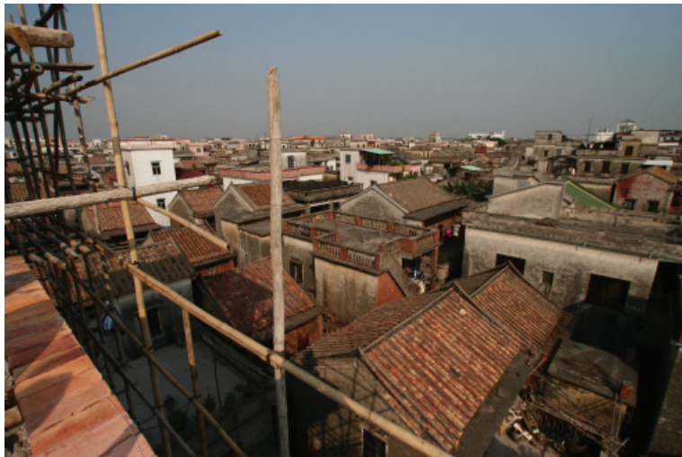
Fig. 160. Residential rooftop. Photograph.
