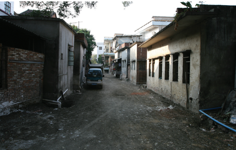
Fig. 353. Canal X after filled with earth and turned into vehicular road. Photograph.
