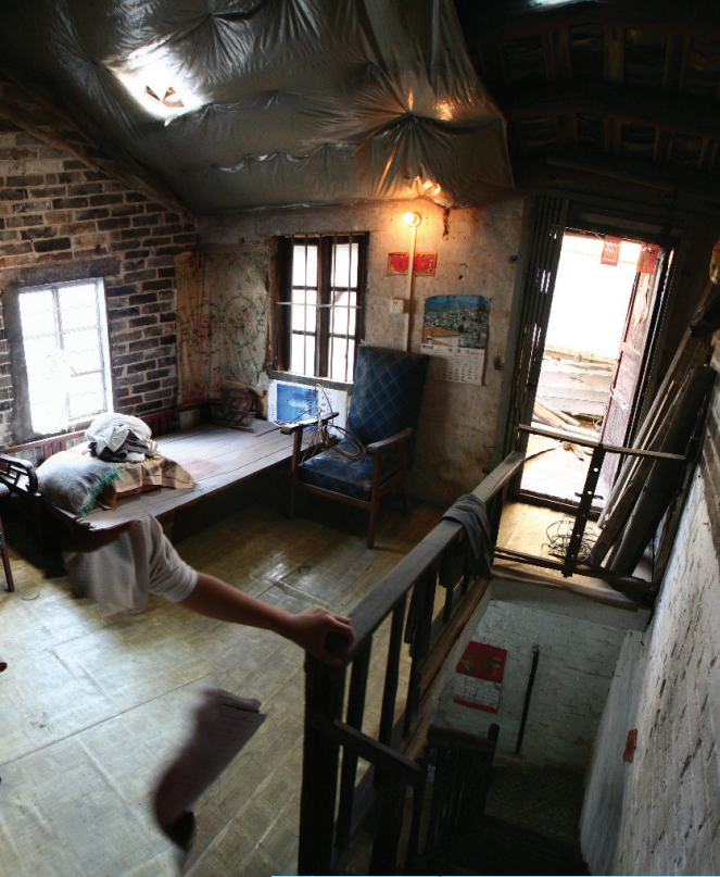
If the mezzanine counted as a separate room, the 56.5m 2 house has three bedrooms.
