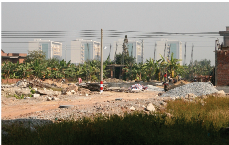
Fig. 85. Dormitory blocks built by village collective.
