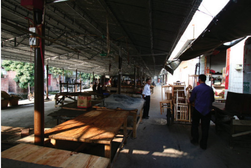
Fig. 181. Open-air sheltered market. Photograph.
