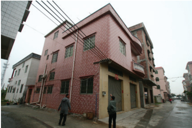
Fig. 188. One-lane vehicular roads around new housing-base houses. Photograph.
