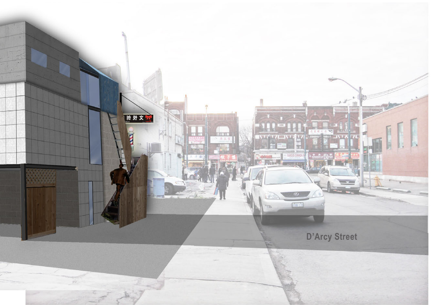
Fig 4.09: Building perspective, looking at the northeast corner.
