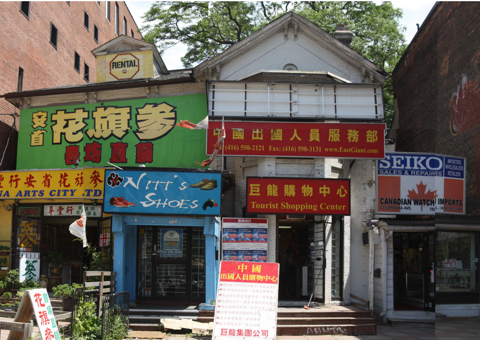
Fig 2.24: Existing façade of the building.
