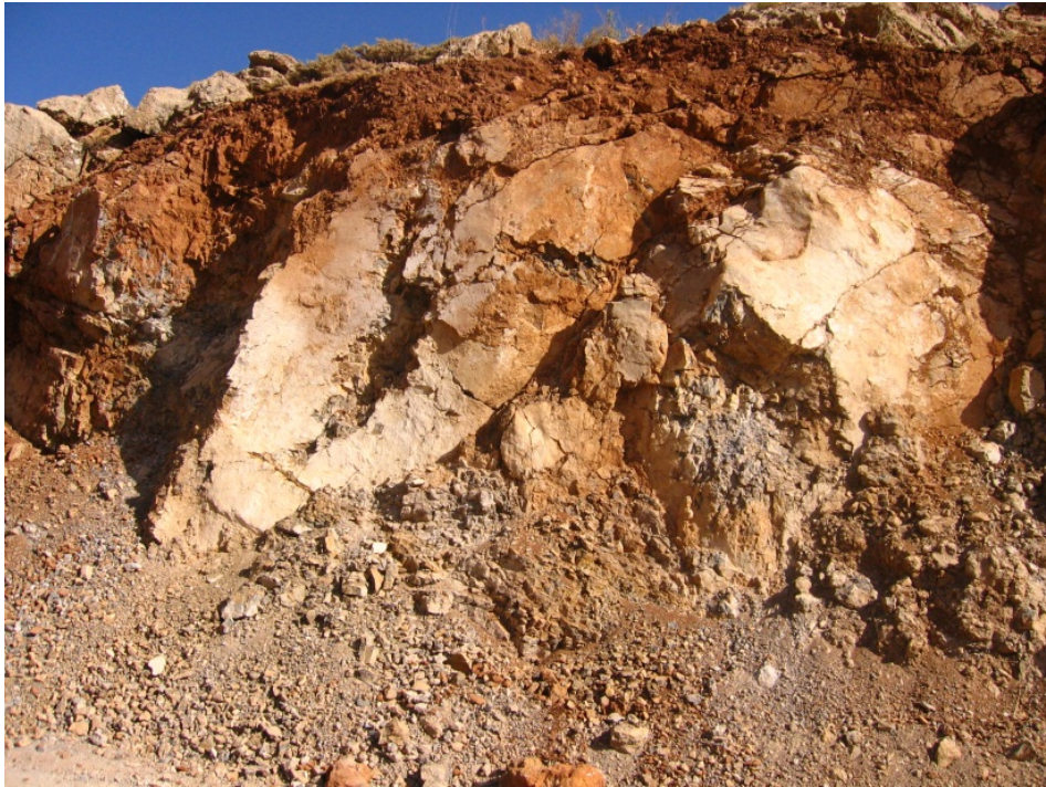
Figure 8-2: Shear fracture on a shear joint surface in limestone from Iran.
