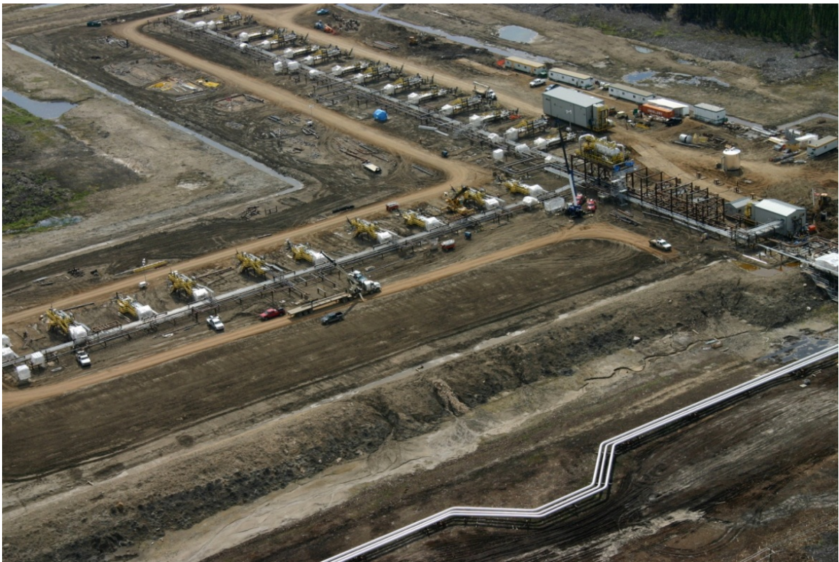
Figure 2-31: SAGD Development, eastern Alberta. Courtesy David Dodge, Pembina Institute.
