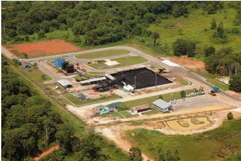
Figure 2-33: Deep Injection Facility for Solid and Liquid Wastes, Duri Oilfield, Indonesia. The black area is a concrete pit for viscous fluids and solids in transit. Duri Oilfield has close to Zero Discharge status.
