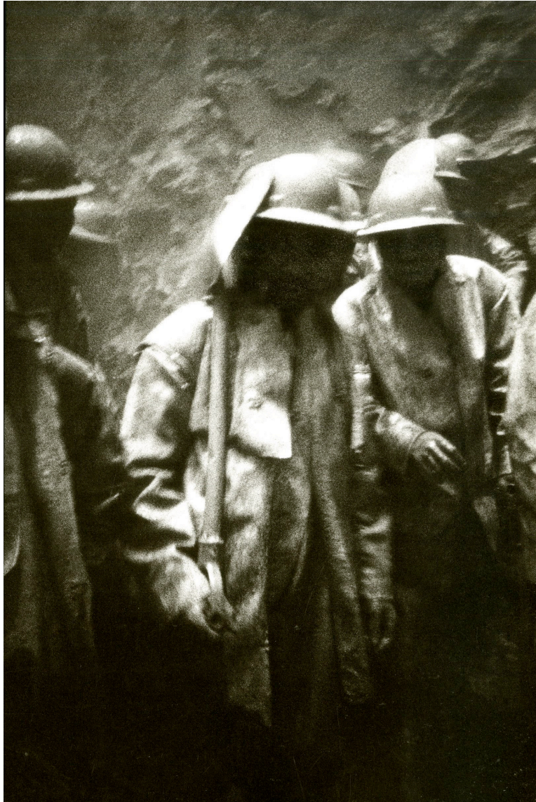
Fig. 36. While the bottom is being blown over with compressed air to uncover misfires, men use shovels to shield their faces from the stinging blast of stone fragments and mud driven through the air at high speeds. President Steyn No. 4 Shaft, Welkom, Orange Free State, January 1970 (Photographer: David Goldblatt).
