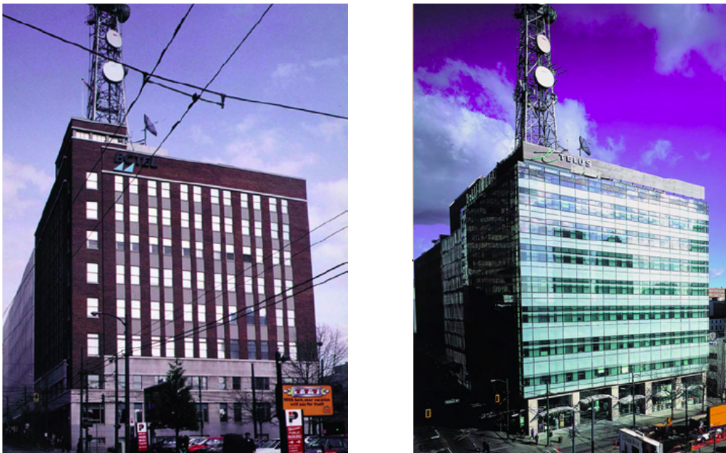
Figure 2.10 William Farrell Telus Building Before and After Retrofit (oikos, 2001)
