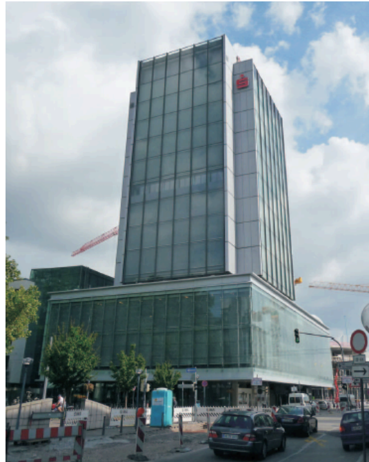
Figure 2.14 Sparkasse Vorderpfalz Post-Retrofit (Ebbert, 2011)
