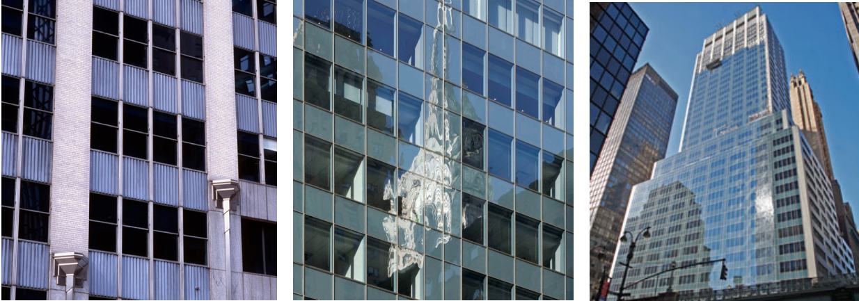
Figure 2.23 100 Park Avenue Façade Retrofit (Zerofootprint, 2010) Left: Pre-retrofit, Middle: Post-retrofit, Right: Mid-retrofit
