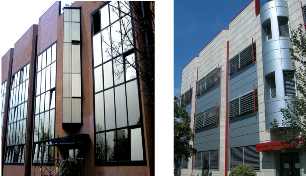
Figure 2.15 ERGO Building Before and After Retrofit (Zerofootprint, 2011)
