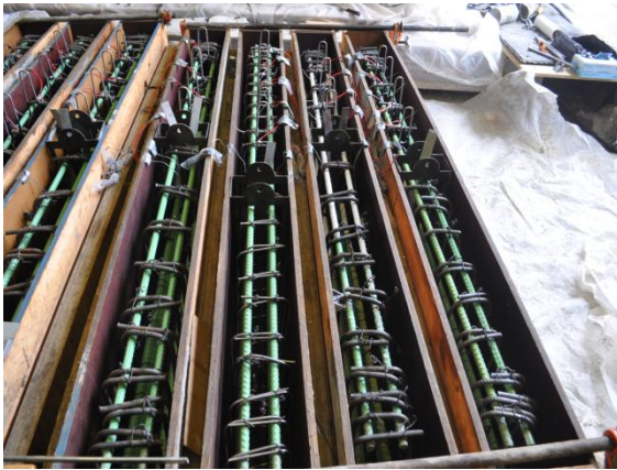
a) One full formwork set consists of four beams
