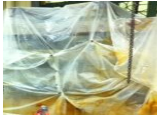
c) Beams covered with plastic sheet to maintain high humidity
