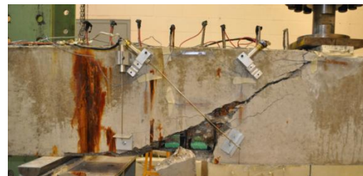
c) High corrosion level beam D6-15%-UR-100
