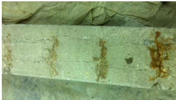
Figure 3.1 Bottom view of corroded shear span (10M-15%-R)
