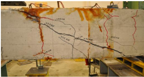
b) Low corrosion level beam 10M-7.5%-UR
