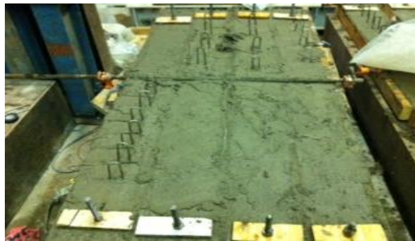
c) One set of four beams after casting
