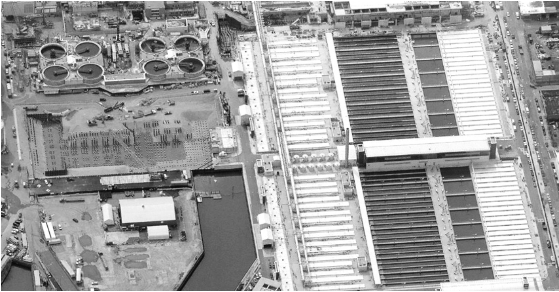
Fig. 2.9 Aerial photograph of New York City's Newton Creek Water Pollution Control Plant illustrating the unpleasant and uninhabitable urban spaces that have been created by the need to facilitate heavily industrialized wastewater treatment processes.
