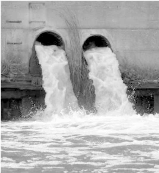
Fig. 1.2 A photograph taken on the East River shows New York City's sewer system spilling untreated effluent into the harbour.
