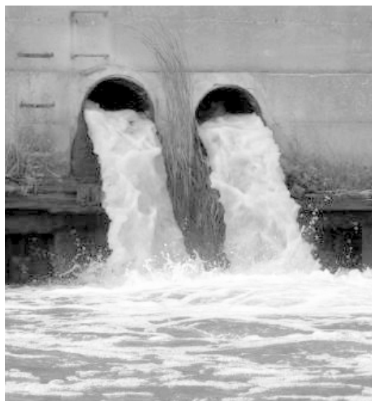
Fig. 2.10 Overtaxed sewers spilling untreated effluent into New York City's East River through combined sewer outfalls.
