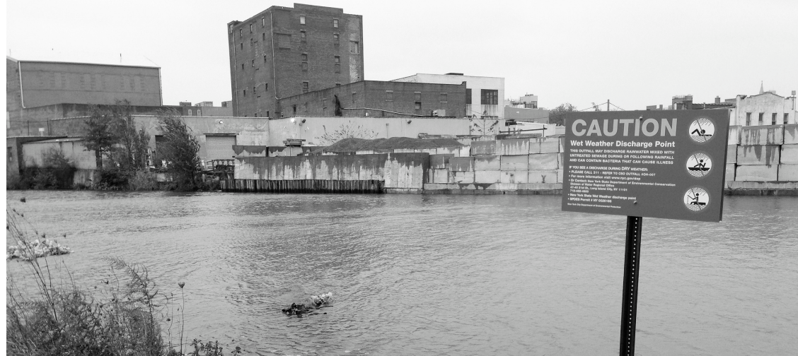
Fig. 6.1 A photograph taken on the banks of the Gowanus Canal shows the present hazards of combined sewer overflow.
