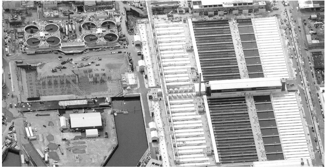
Fig. 1.4 New York City's largest sewage treatment facility, the Newton Creek Water Pollution Control Plant.
