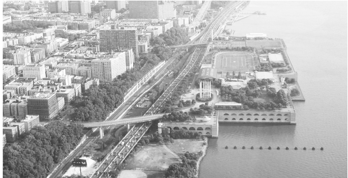
Fig. 3.5 An aerial photograph of New York City's North River Wastewater Treatment Facility illustrates how the infrastructure was made an accessible and integrated element of Manhattan's public waterfront by its ability to function as a public park.
