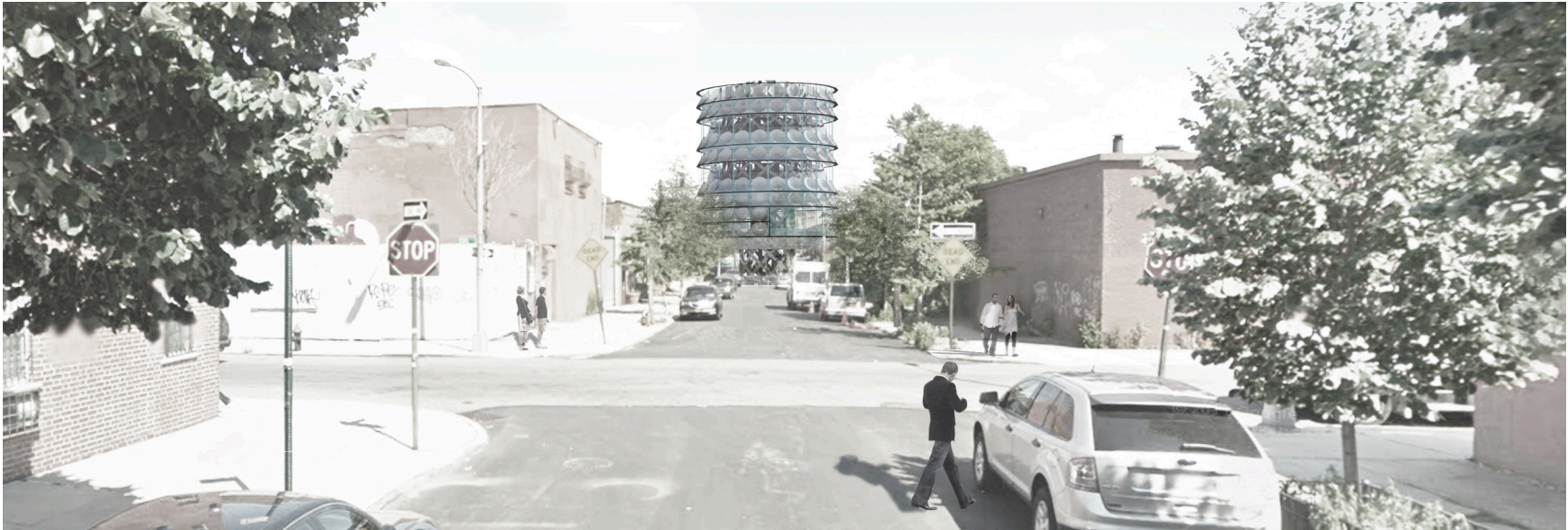
Fig. 5.17 A down Degraw Street shows an iconic “Living Machine” tower positioned at its terminus.
