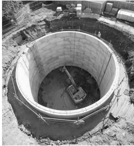
Fig. 1.3 A photograph of a typical cistern designed to intercept and store excess sewage that overflows into urban waterways.
