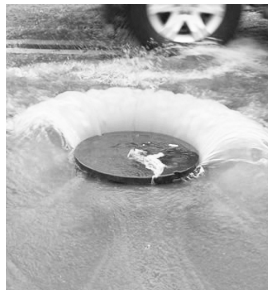
Fig. 2.11 Overtaxed sewers in midtown Manhattan backup through a manhole spilling untreated sewage into the streets.
