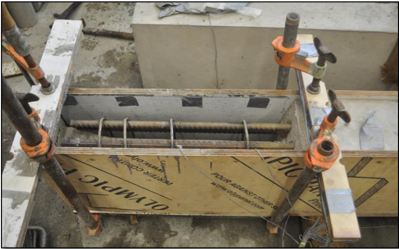
Figure 3.18 The formwork for repairing the beams
