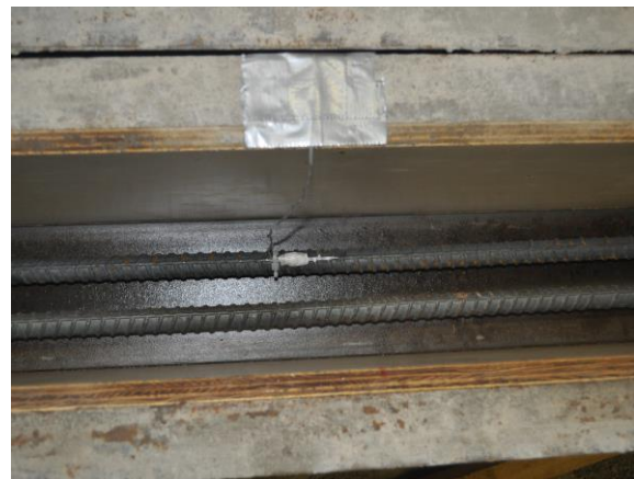
(b) Strain gauge installation
