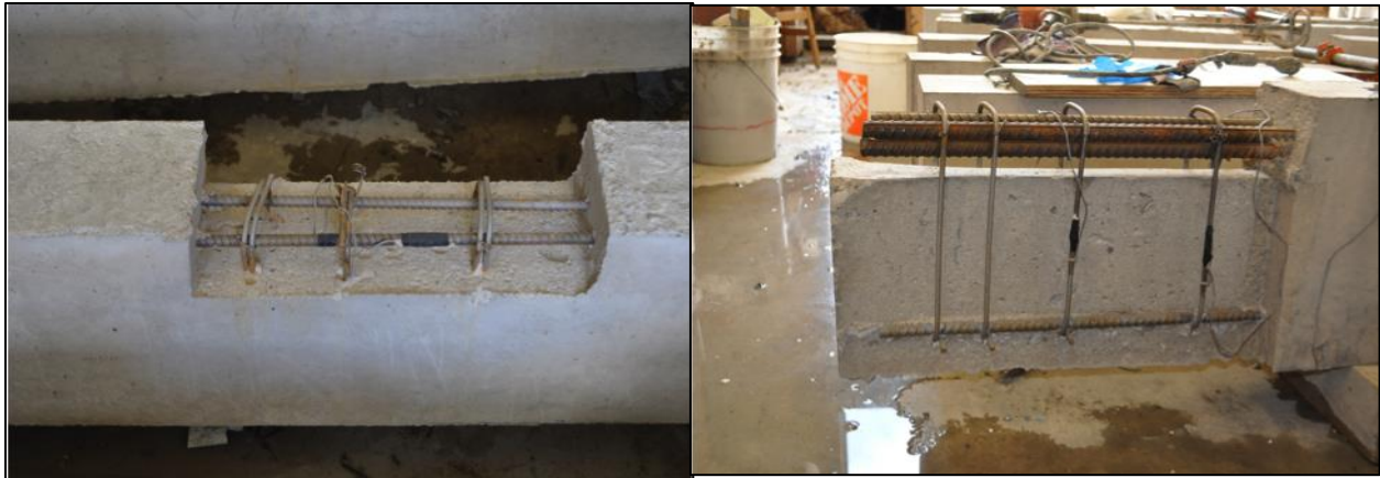
Figure 3.16 Beams configuration before repair
