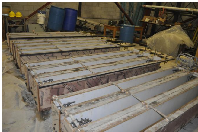
(a) Beam formwork
