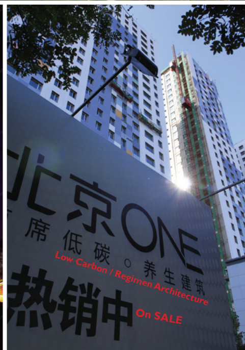
0.1.15 Beijing ONE under construction, 2011
