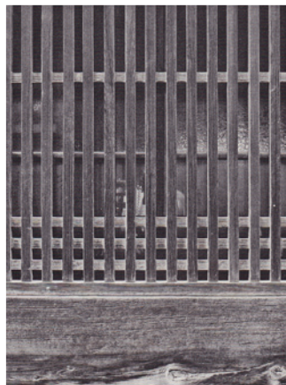
2.1.7 Vertical mullion window in Imai cho, Nara, Japan.
