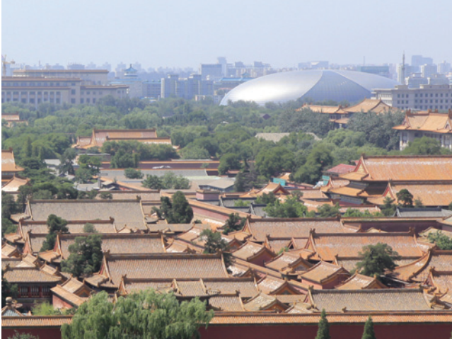
I.1.25 National Grand Theatre of China by Paul Andreu protrudes out from the uniformed historic fabric of the Forbidden City.
