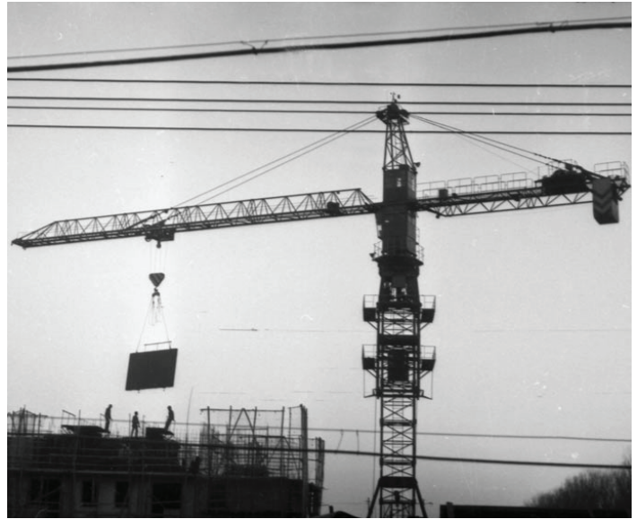
I.1.12 Slab construction, 1978
