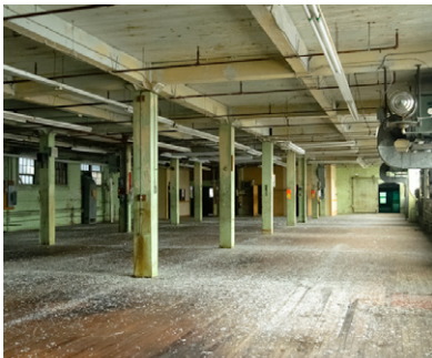
fig. 3.63 interior mill conditions
