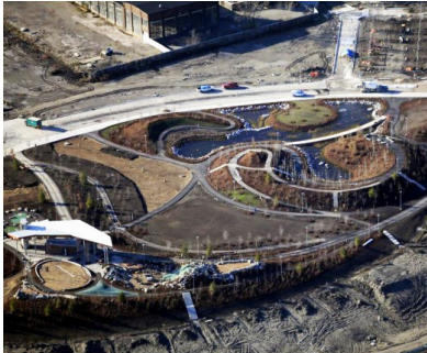
fig. 3.55 landscape in progress
