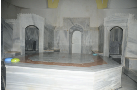
Fig.3.19. Belly stone in the men's hamam. On the background, doors lead to the ablutions zone, on the left and right sides.
