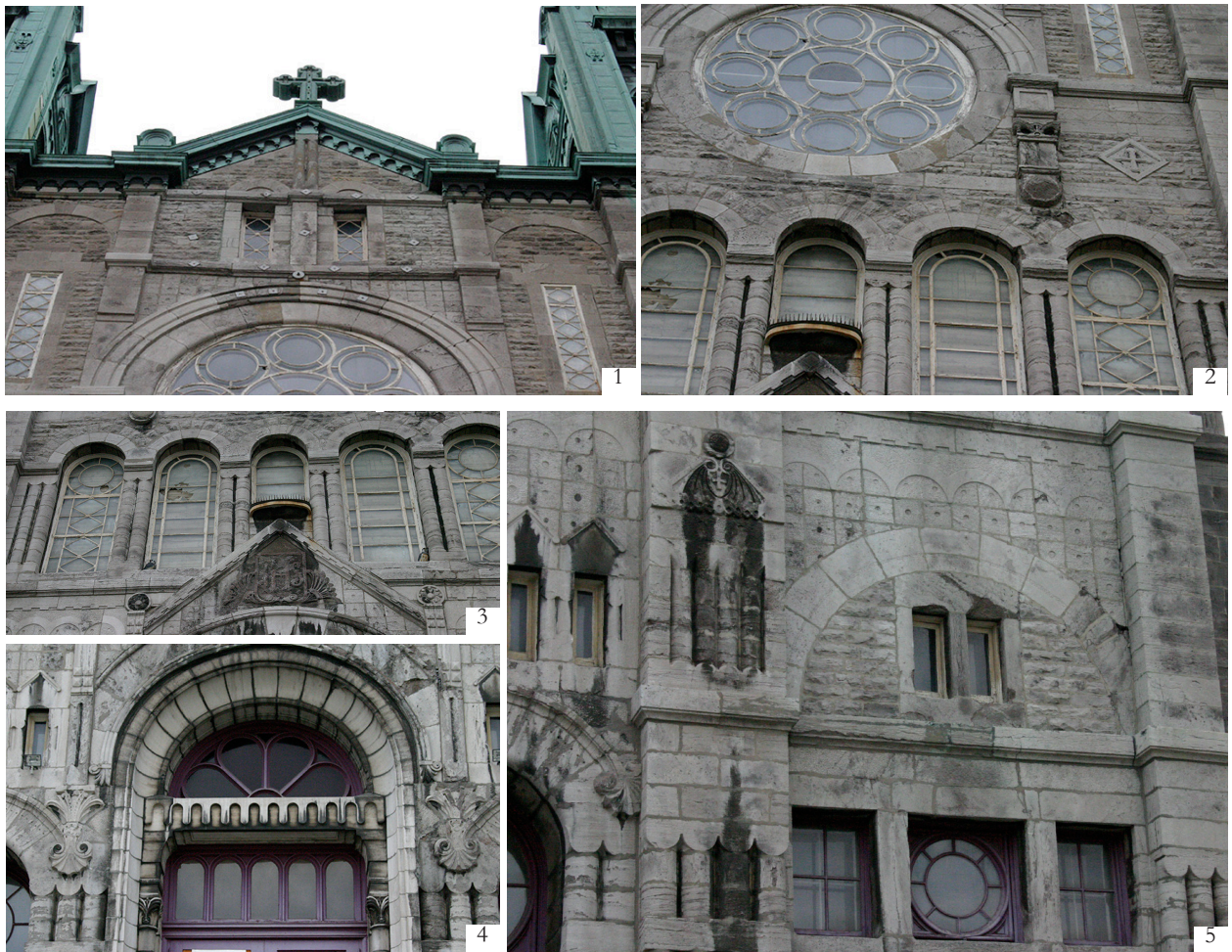
Fig.3.34. Current conditions of the façade.
