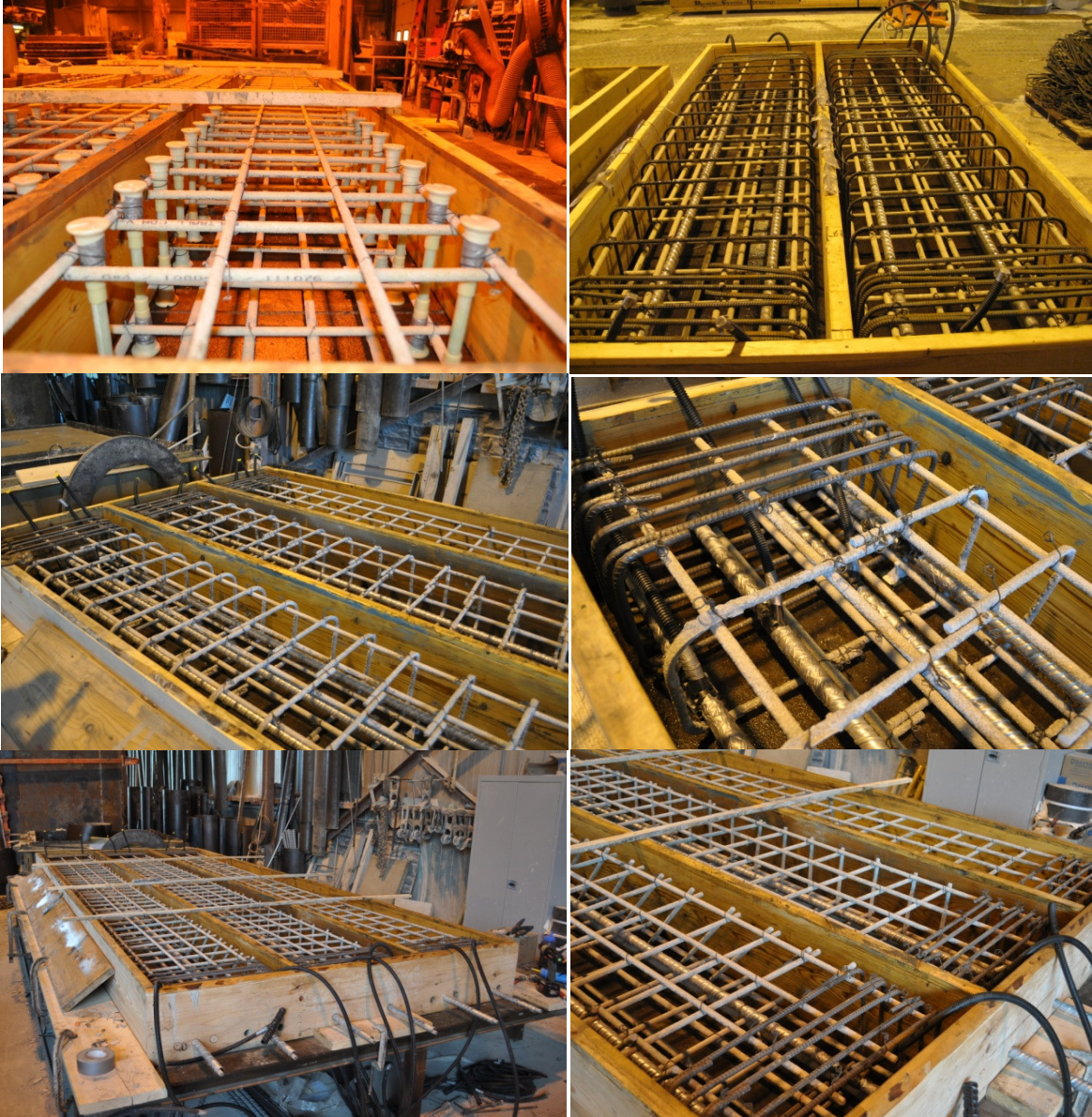
Figure 3.12 - Completed reinforcing cages in wooden formwork
