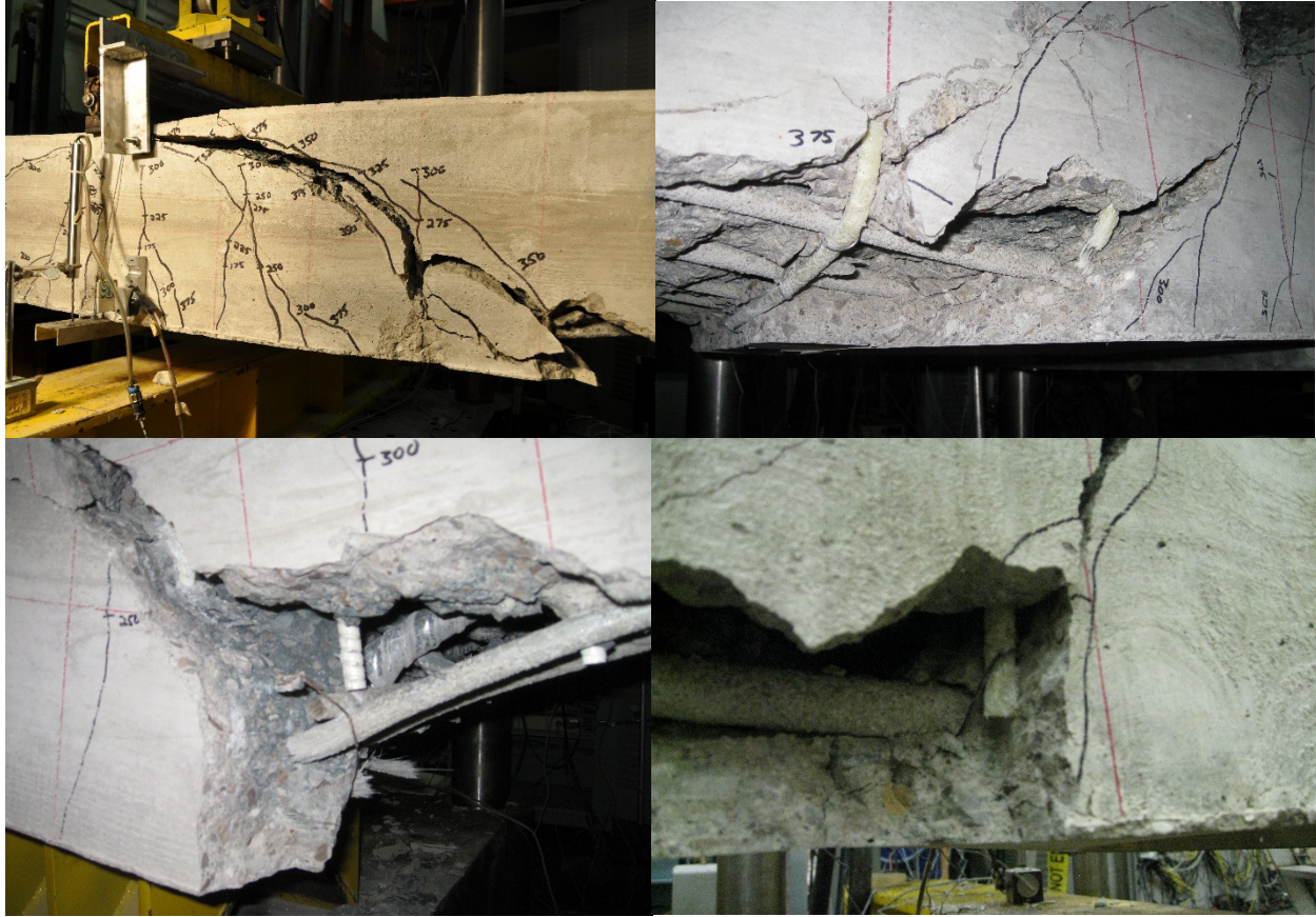
Figure 4.15 - Typical shear failures for Phase II slabs (Clockwise from top left: critical shear crack; failure of C-shaped stirrup at bend location; U-shaped stirrup pullout failure; failure of anchor head)
