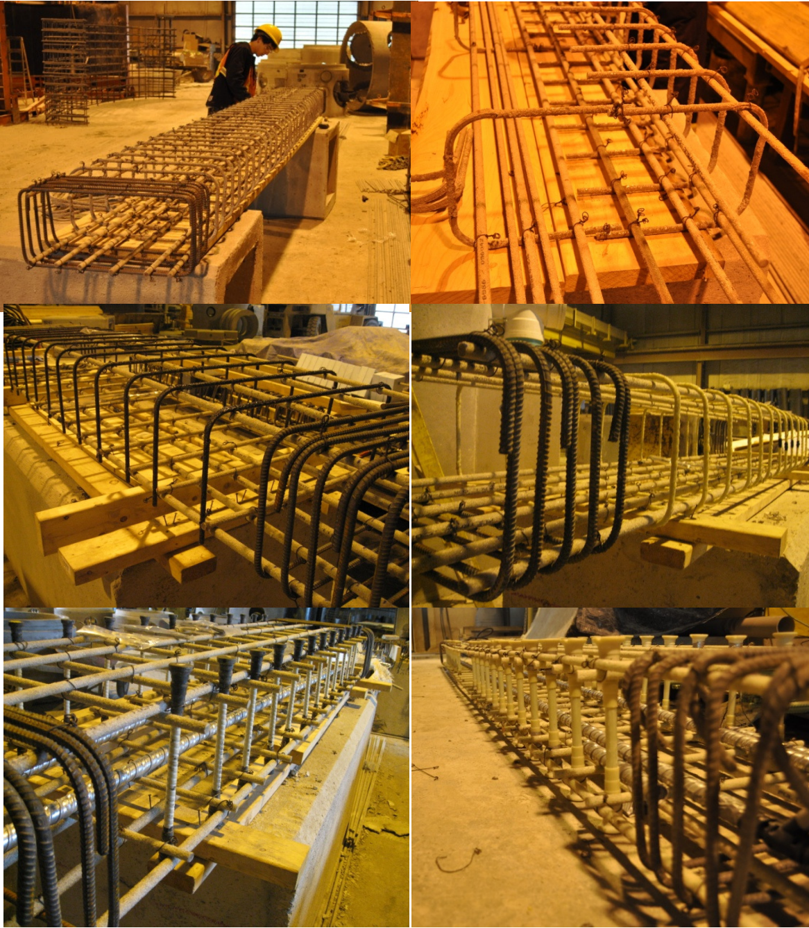
Figure 3.11 - Construction of reinforcing cages with various types of shear reinforcement
