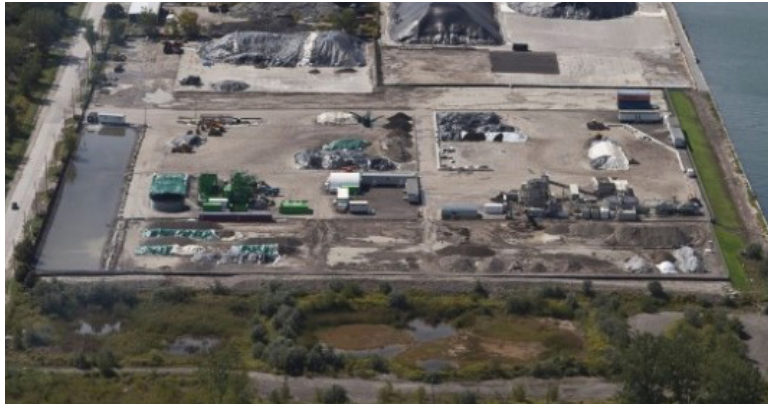
fig. 2-67 Port Lands Soil Recycling Pilot Facility
