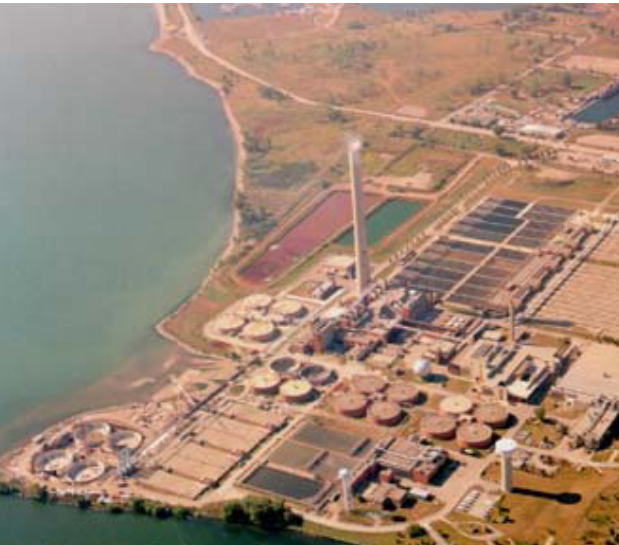
fig. 2-42 Sewage Treatment Plant
