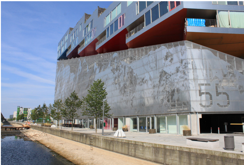
fig. 4-34 Canal-side 'Mountain' Dwellings
