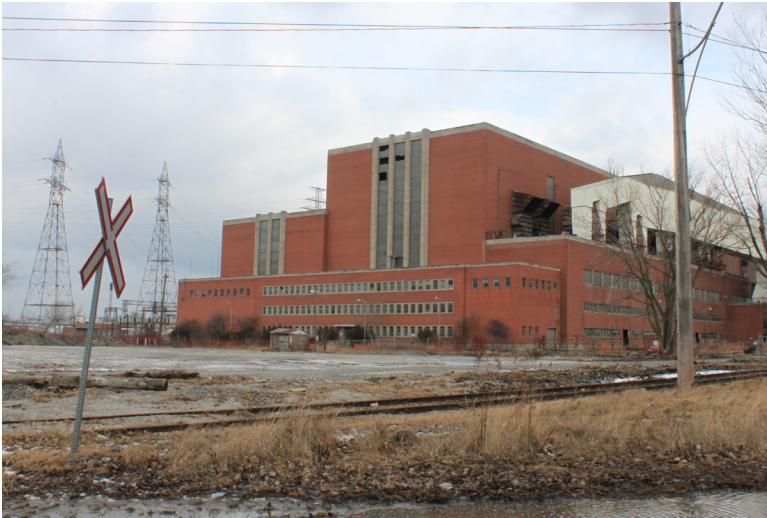
fig. 3-32 Hearn Power Generation Plant
