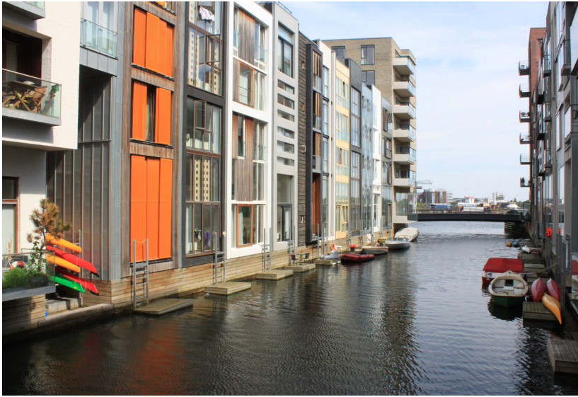
fig. 4-27 Canal-side duplex housing
