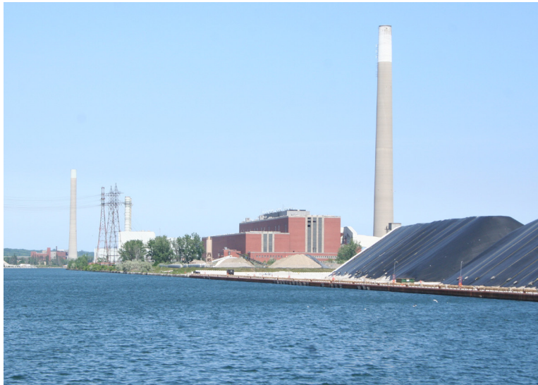
fig. 2-57 Shipping Channel + the Hearn Generating Plant
