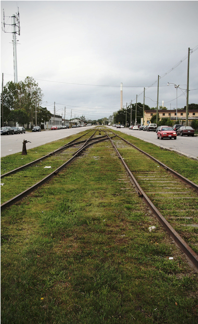
fig. 2-35 Obsolete industrial rail infrastructure on Villiers St.
