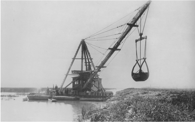
fig. 2-29 Dredging of the Marsh for the Port Industrial District
