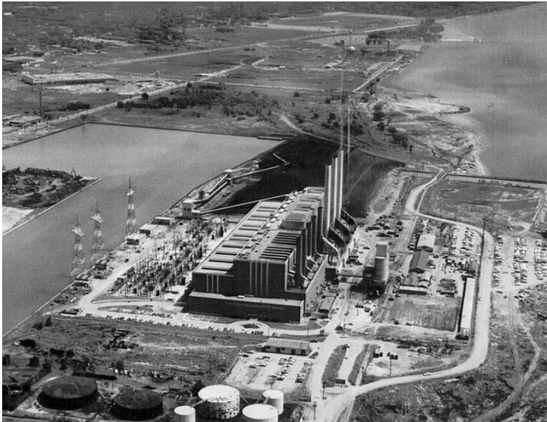
fig. 2-30 The Hearn power generation plant
