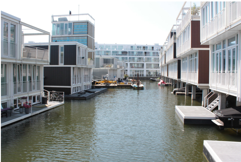
fig. 4-11 Self-built water housing
