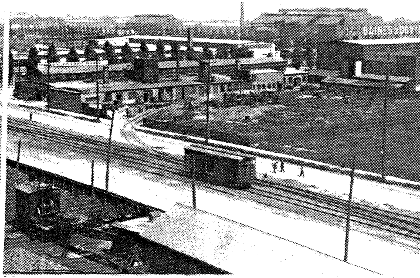
Munitions Street is complete, Bond Engineering and Baines and David on the west, Canadian Ice Machine and Disher Steel on the east side.
