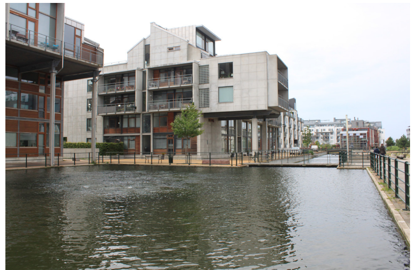
fig. 4-42 View from canal
