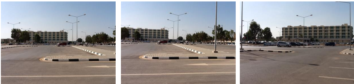
Figure 5.17: Parking and paved walkways
