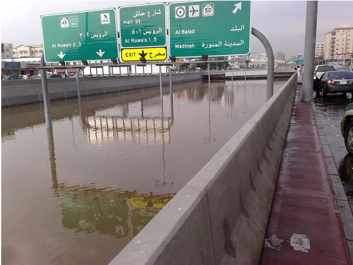
Figure 1-1 Flood in the canal of King Abdullah Road, Jeddah, Saudi Arabia, November 2009.
