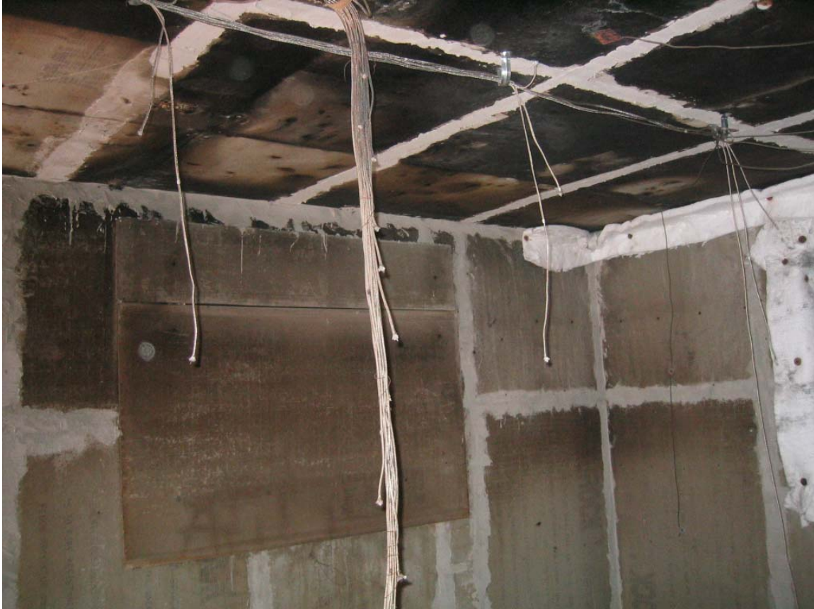
Figure 3.10: Thermocouples Positioned at Ceiling, 8" (203 mm) and 16" (406 mm) Down from Ceiling for Third and Fourth Experiments
