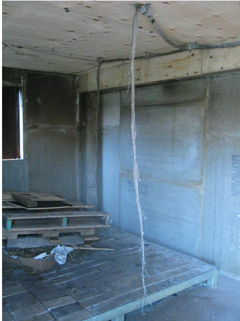
Figure 3.9: Thermocouple Positions in Rake 2 and Ceiling Hangars
