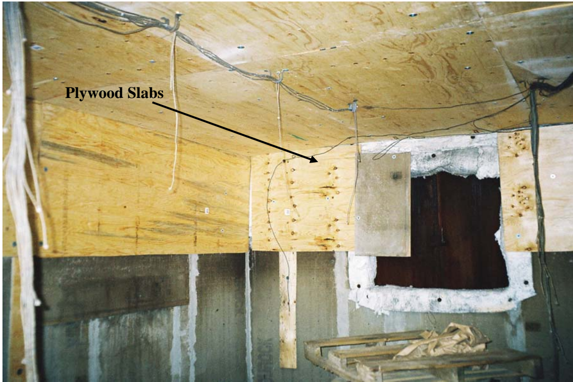
Figure 3.13: Burn Room Interior Wall Construction, November 25, 2004
