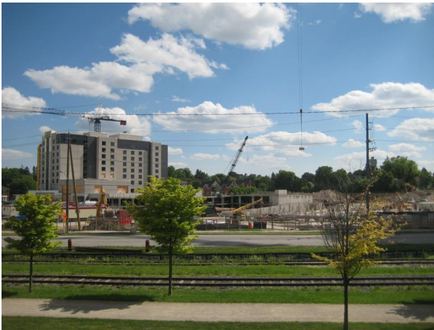
Figure 12. Construction of the Barrel Yards development located near Uptown Waterloo.
