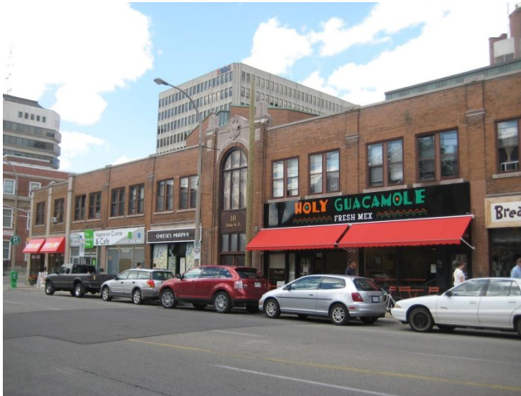
Figure 11. An area of revitalization in Downtown Kitchener located on Duke Street between Queen and Frederick Streets.
