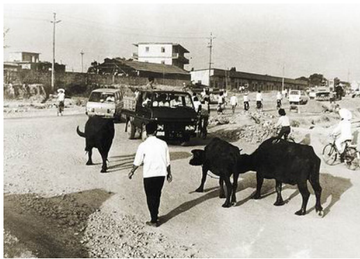
^ Figure 1.5 Transformation of Shenzhen SHENNAN ROAD 1983
