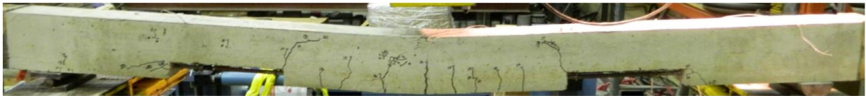
Figure 4-32: Crack pattern for specimen 5
