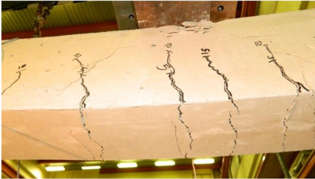
Figure 4-72: Bottom crack in specimen 11
