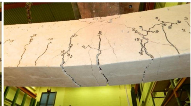
Figure 4-65: Bottom crack in specimen 10
