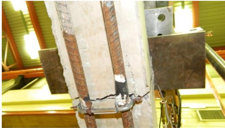
Figure 4-23: Mid-span crack for specimen 4
