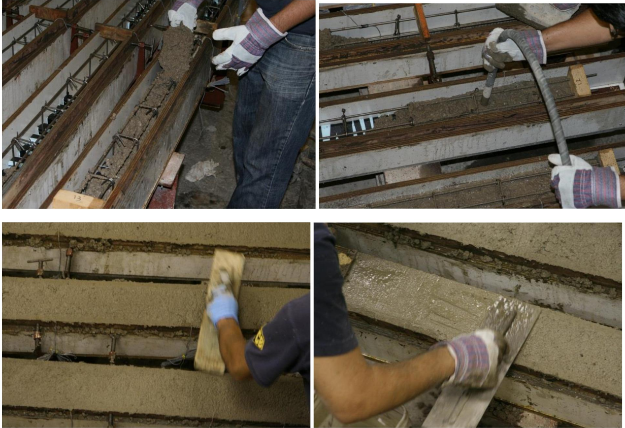
Figure 3-10: Concrete of casting, vibration and smoothing the surface
