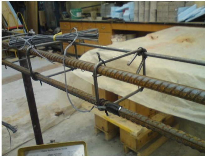
Figure 3-9: Strain gauges installation
