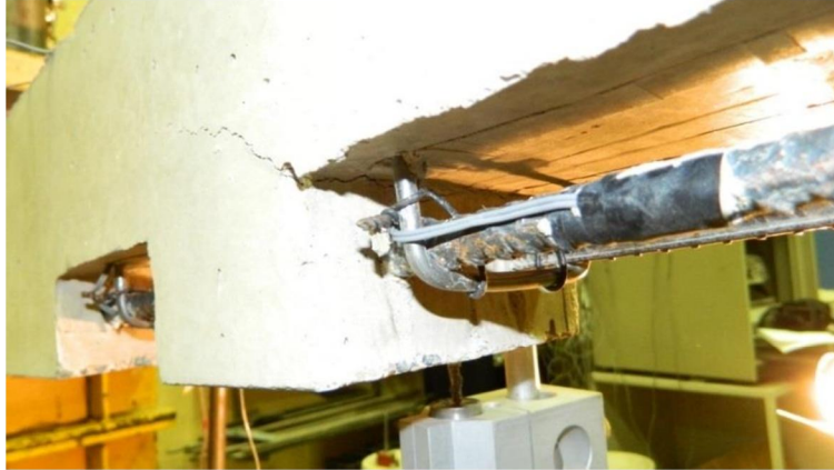
Figure 4-73: Corner crack propagation
