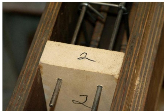
Figure 3-4: Form work preparation
