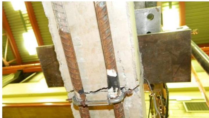
Figure 4-9: Average crack wide for specimen 2
