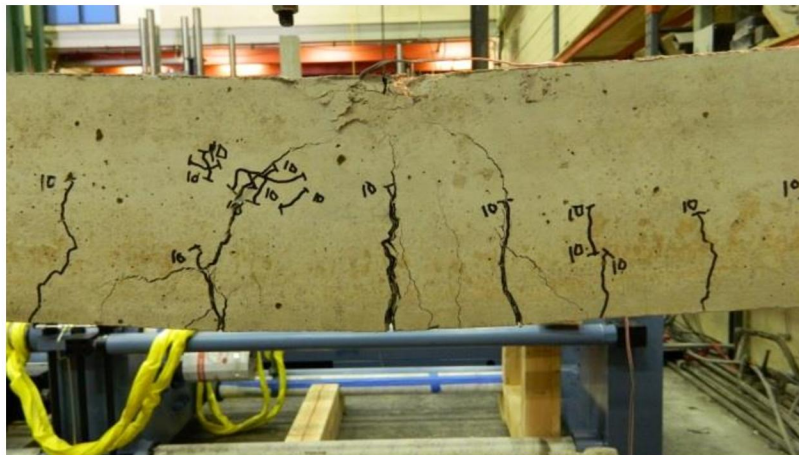
Figure 4-28: Flexural crack for specimen 5
