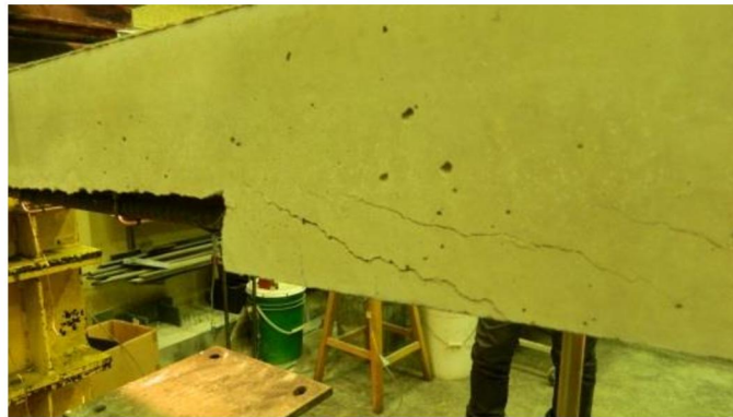
Figure 4-86: Pull out crack for specimen 13
