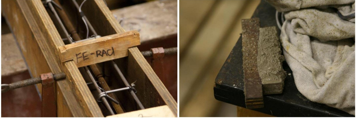
Figure 3-5: Wooden support for hanging the cage in concrete casting
