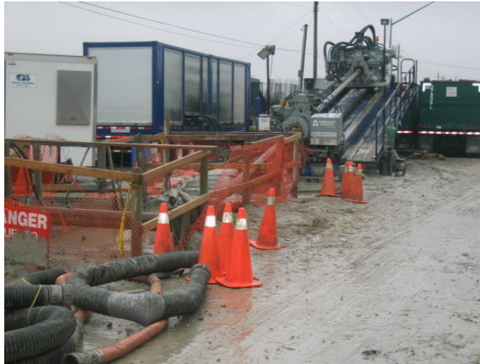
Figure 5: American Auger DD-1100 Set up in the field
