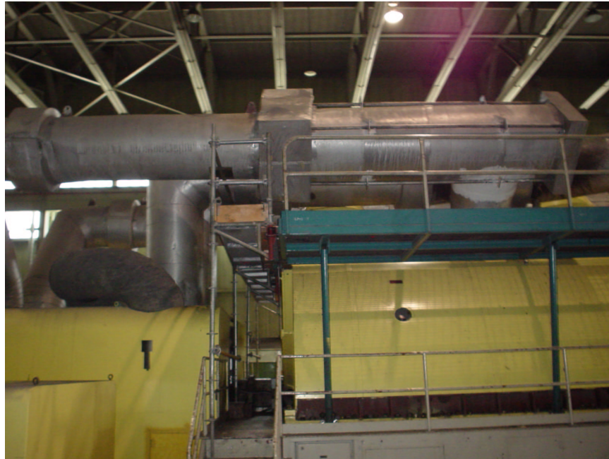
Figure 5.7: Low-pressure section of Naticoke turbine
