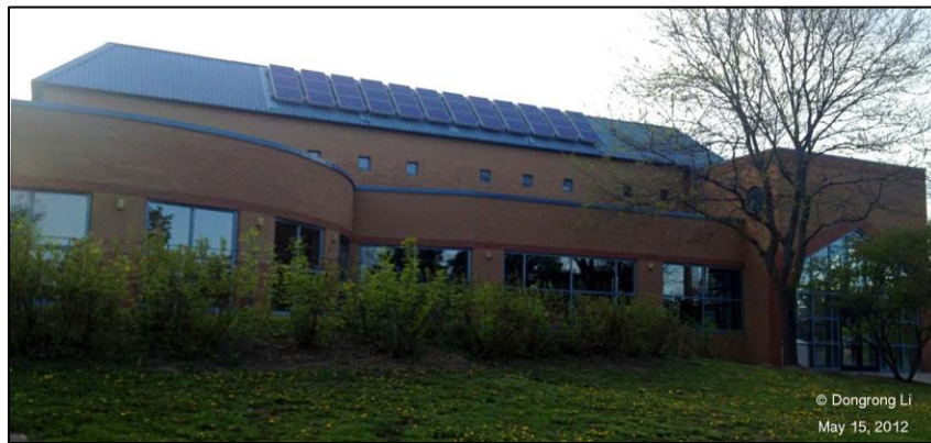
Figure 2.5 - Solar panels on the FED Hall rooftop
