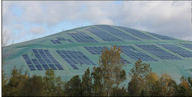
Figure 6.1 - A landfill site on the outskirts of Atlanta, Georgia covered 10 acres of land with plastic solar panels (Snedden, 2011)
