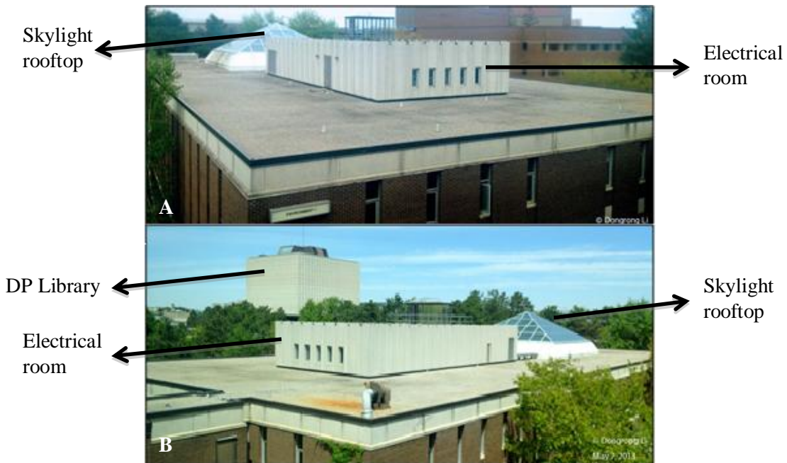
Figure 3.3 - Pictures of the EV1 and DP Library roofs
