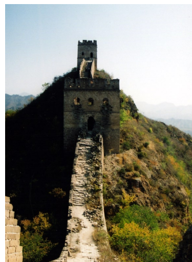
Fig. 1.23 A section of the wall without much renovation.
