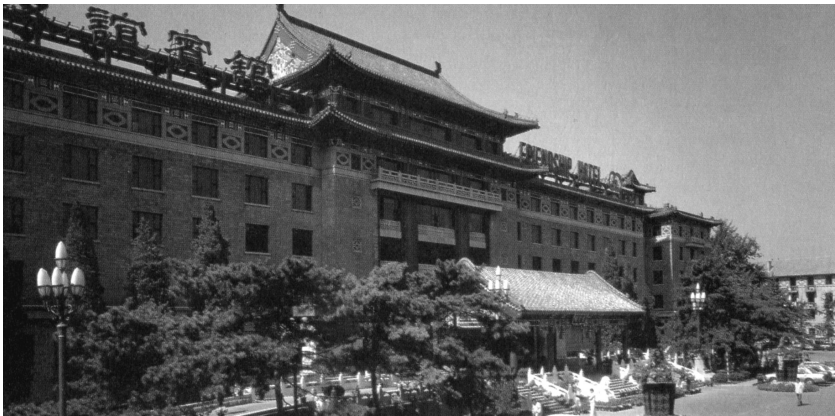
Fig. 8.26 The Friendship Hotel was built in 1955. The 260,000 sq. m building contains a 1200-seat auditorium, a 1000-seat dining hall and 1900 guest rooms. The 7-storey building is considered one of the masterpiece of "big roof" projects. It contains Chinese roofs, pavilions, podiums, and traditional motifs for decorations.
