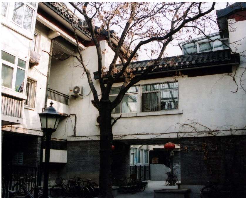
Fig. 8.39 Semi-private courtyard of Wu Liangyong's Juer Hutong project.
