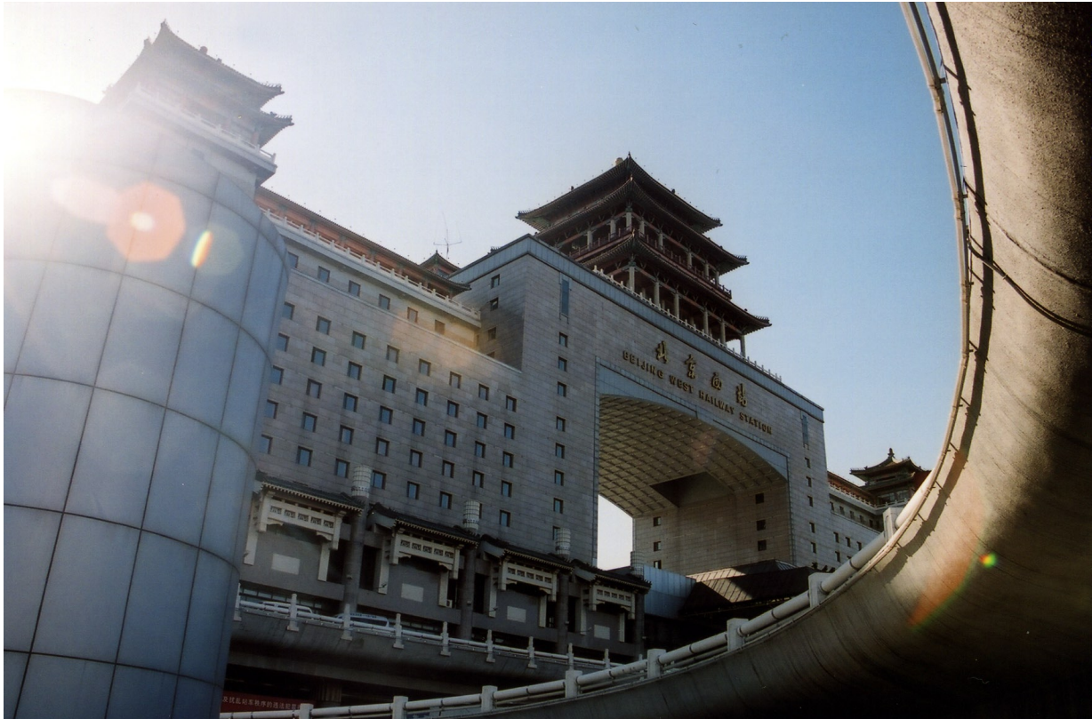
Fig. 1.38 Beijing West Railway Station exemplifies the Chinese post-modernist movement in the early 1990s.
