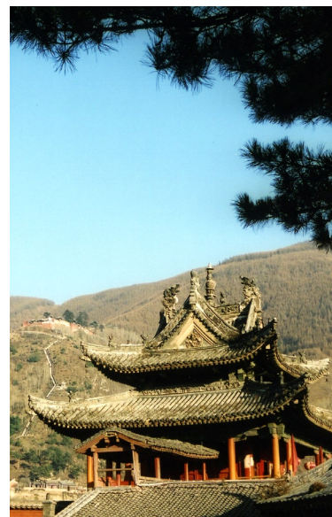
Fig. 3.23 A temple entrance tower at Taihuai.
