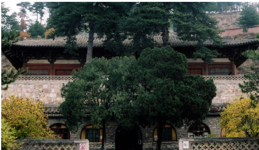
Fig. 3.28 The cave-dwelling like chambers of the intermediate level and the Foguang Main (East) Hall on the upper level.
