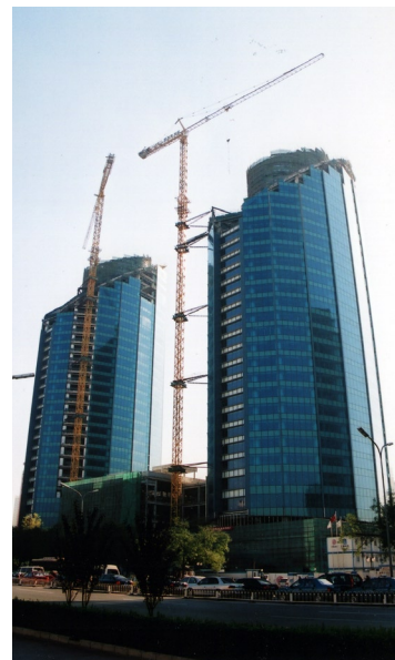
Fig. 5.78-5.79 Many new buildings are under construction in the CBD area.
