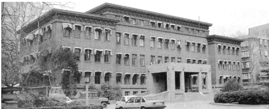
Fig. 8.22 Department of Foreign Affairs of the Republic government (1934), Nanjing, designed by Tong Jun and Zhao Shen.
