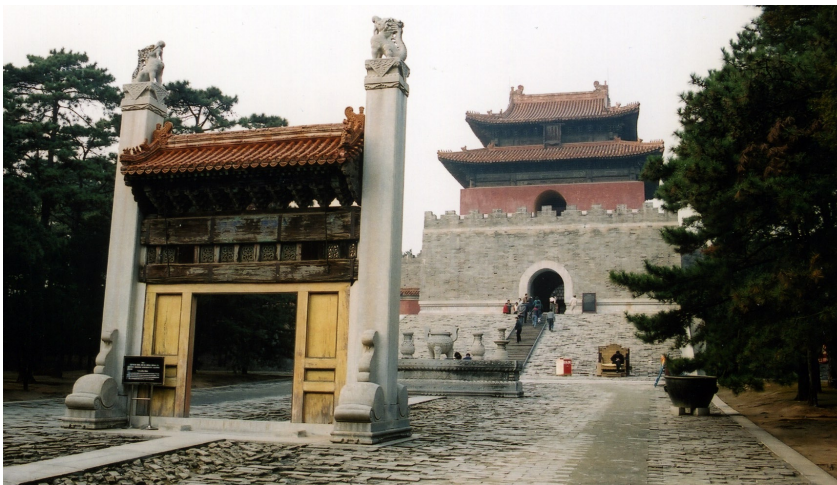
Fig. 5.64 The main courtyard of the Yin World at Qianlong's tomb. The self-standing stone gate represents the official entry into the world of the dead, while the stone counter stands in midway between the gate and the mausoleum.
