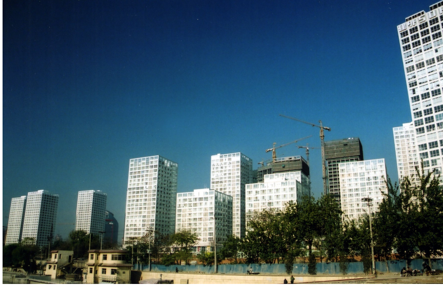
Fig. 7.14 Japanese architect Riken Yamamoto took great care with orientation of the towers at Jianwai SOHO to maximize the amount of sunlight each unit receives.
