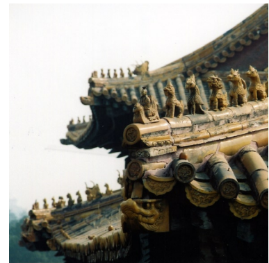
Fig. 1.16 Typical roof decorations made of yellow glazed tiles on the imperial palaces.
