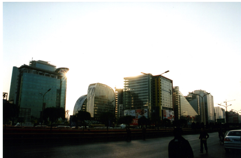
Fig. 7.16 Most of the futuristic buildings at Zhongguancun are close to completion.
