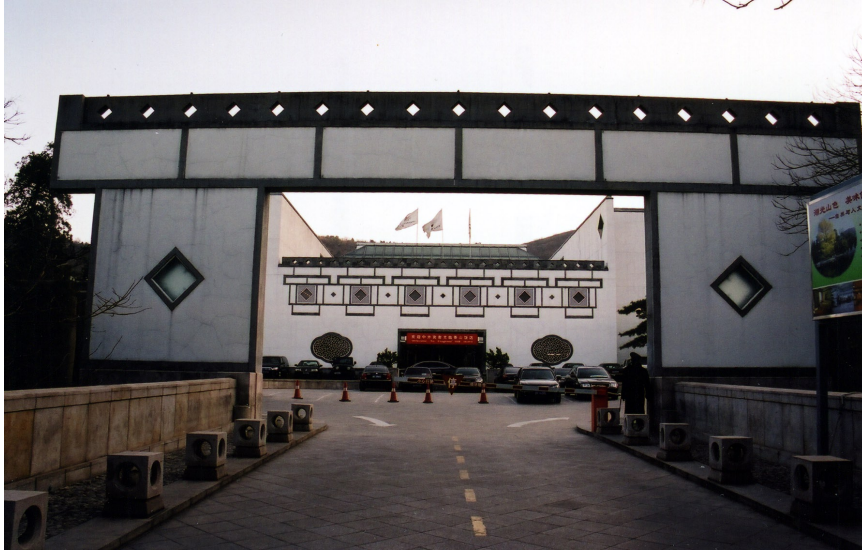
Fig. 7.35 The front entrance of the Xiangshan Hotel.
