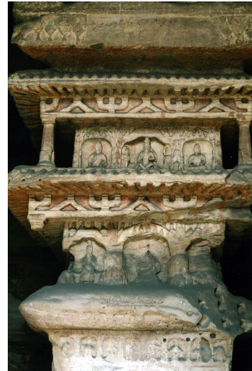
Fig. 8.1 Built by a non-Han emperor in the fifth century, the Yungang Buddhist Grottoes present a number of early Chinese architectural elements. This column at Grotto #2 depicts a multi-storey building, including an early form of dougong brackets.
