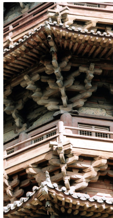
Fig. 3.37 Dougong brackets of the Fogong Temple Wooden Pagoda, Yingxian.
