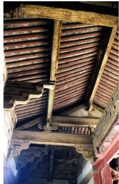
Fig. 5.70 The exposed structure of the Shanmen of Dule Temple.
