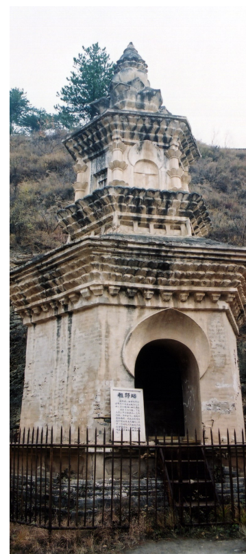
Fig. 3.30 The Chief Priest Tower adjacent to the Main (East) Hall of the Foguang Temple, Wutaishan.
