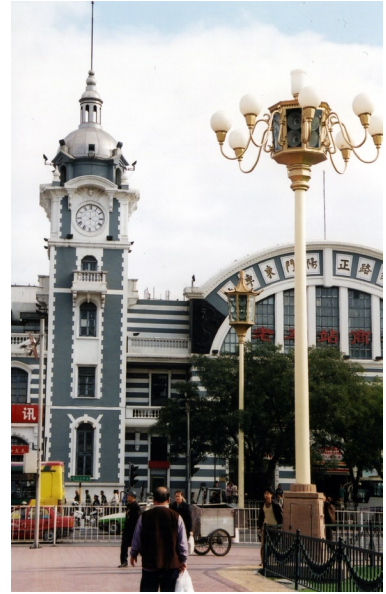
Fig. 5.5 The former Front Gate Railway Station.
