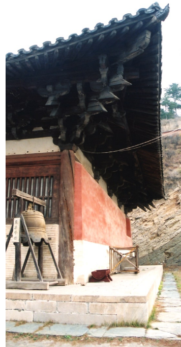
Fig. 8.16 The eaves and the corner dougong of the Foguang Temple Main Hall, Wutaishan.
