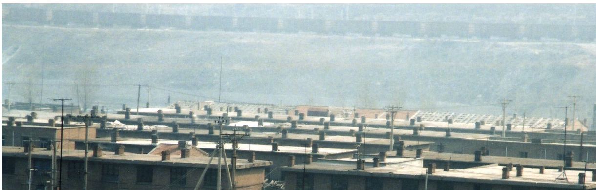
Fig. 3.51 The worker houses in the town of Yungang and the coal freight carts at the back.
