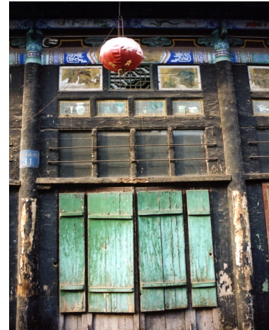
Fig. 3.14 A traditional window opens to the Ming-Qing Street at old Pingyao.
