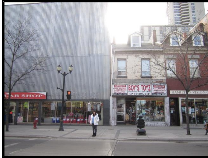
(Figure 13: My dollar Shop, located within the International Village BIA, looking north, Example of Very Poor Building Conditions)
