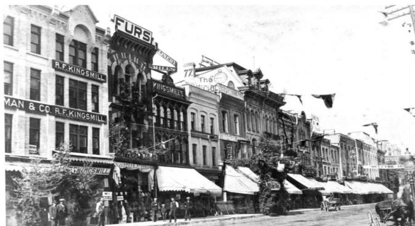
Fig. 4-9: North block of Dundas street, date unknown. Newer architectural styles exist as the eye is drawn to the right. The awnings are also among the most notable features of the buildings. Source: Archives and Research
