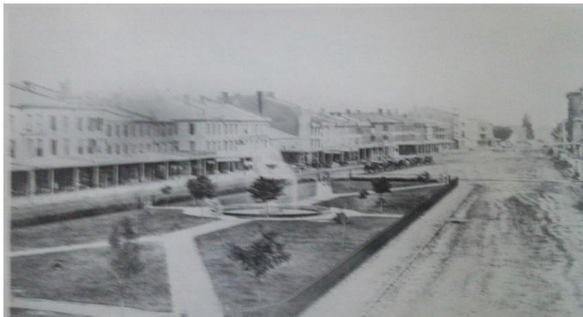
Fig 5-5: Gore Park and King St E, picture taken after the street was macadamized in 1862. Source: Weaver, 1982
