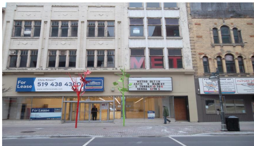
Fig. 4-16: Dundas Street. A number of buildings remain vacant, thereby further delaying much needed maintenance. Source: Author
