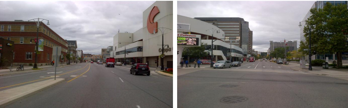
Fig. 6-9: Copps Coliseum and surrounding streetscape along York Blvd (a) and Bay St, looking south (b).
