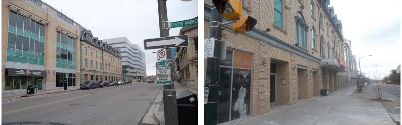
Fig. 6-12: Budweiser Gardens streetscape: a) along Talbot St; b) along Dundas St facing west. Sources: author
