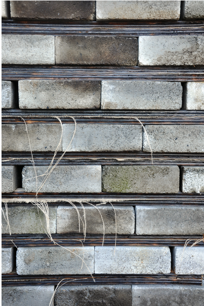
Pyre's Construction Fig. 5.9
