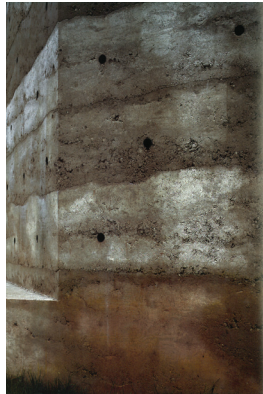
Exterior Detail Fig. 4.29
