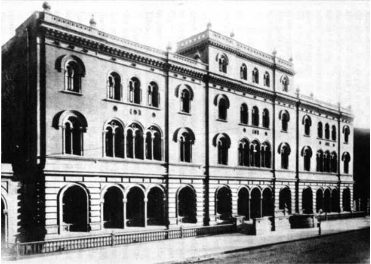
State of the Astor library building as it was when abandoned by the NYPL in 1911.
