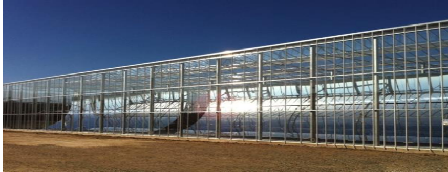
Figure 48 CSP glasshouse (Source: glass point Co. website glasspoint )
