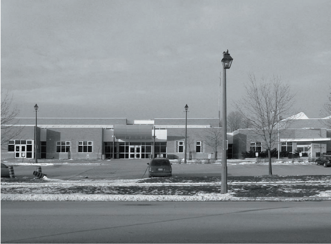
Figure 2.57 Bayview Hills Community Centre Entrance
