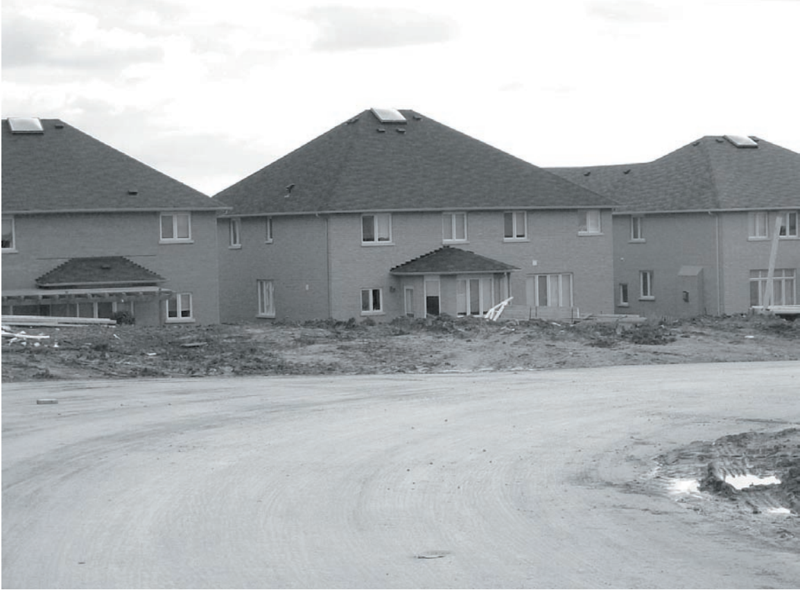
Figure 2.42 On the Senator Homes Construction Site.
