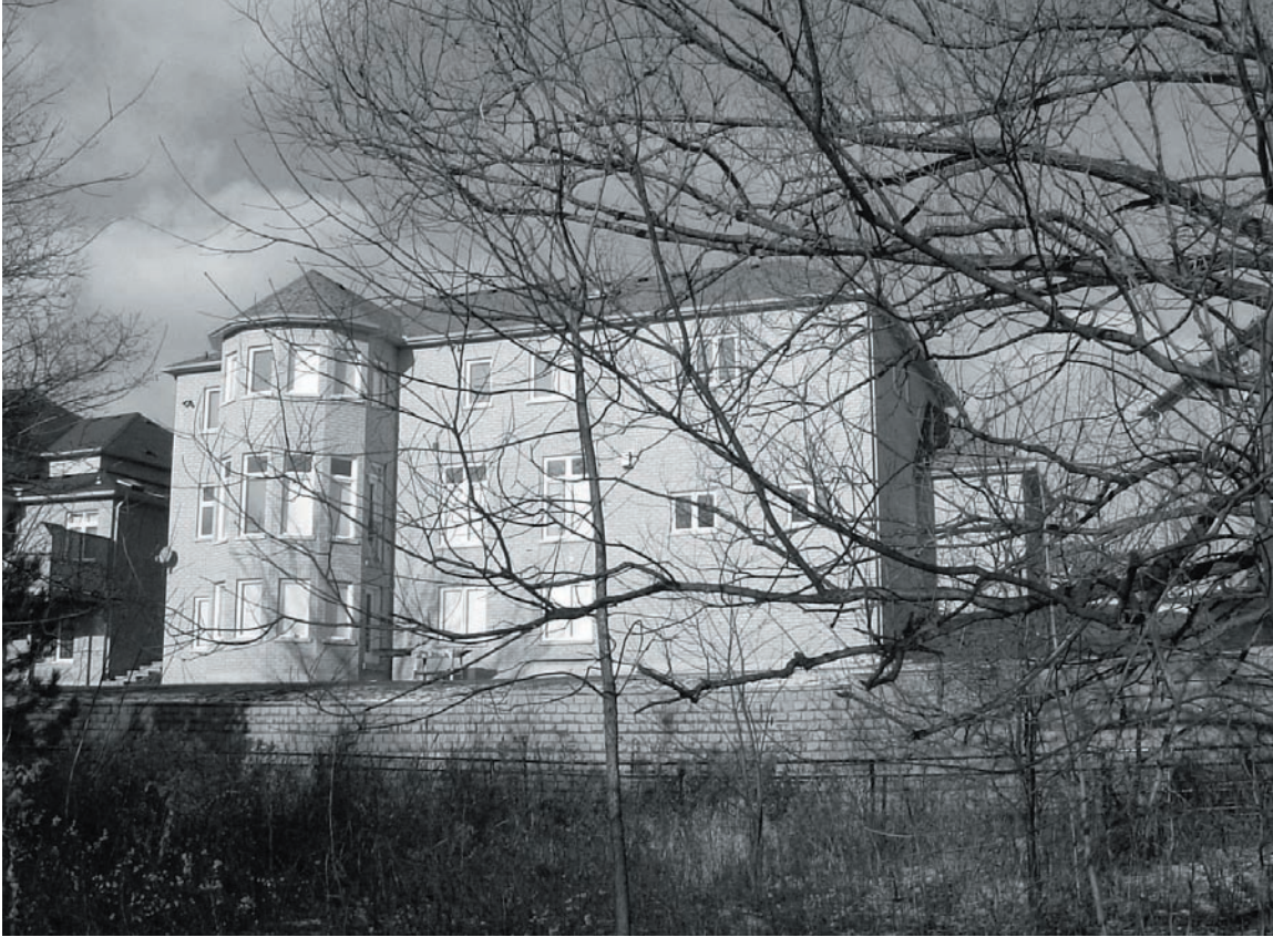
Figure 2.44 Looking at Large House from East Beaver Greenway.
