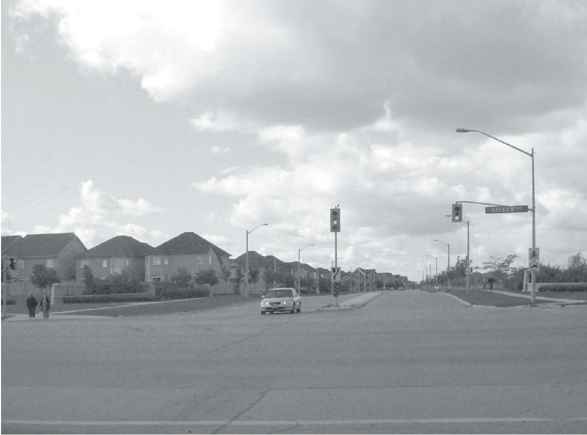
Figure 2.17 Intersection of Bayview and Highway 16.
