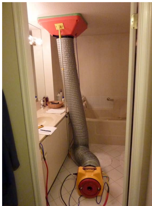
Figure 6-8: Typical Powered Flow Hood Apparatus
