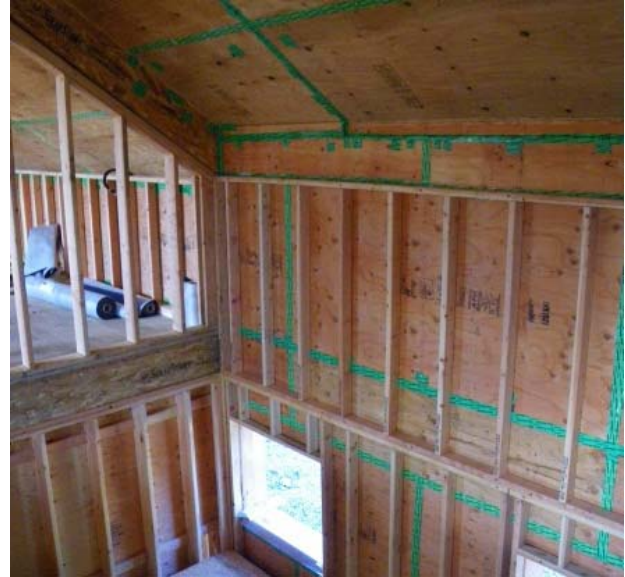
Figure 4-3: Interior plywood sheathing of pre-fabricated wall panel sealed with tape to provide the air barrier. (Photo courtesy of RDH.)
