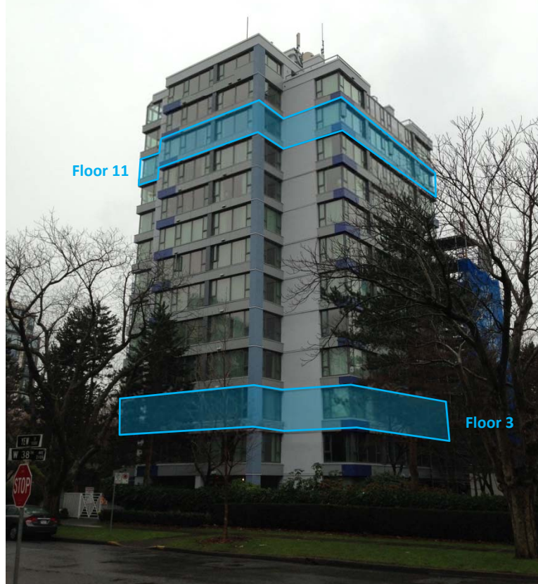
Figure 10-25: Image of North and East elevations of the case study building showing surrounding trees that provide local shielding with respect to wind
