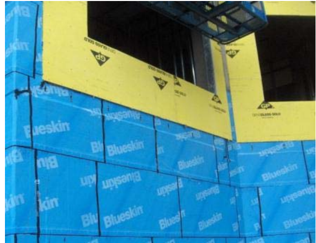
Figure 4-5: Exterior adhered sheathing membrane providing air barrier. (Photo courtesy of RDH.)
