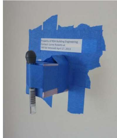
Figure C-2: Photo of typical CATS installation using extruded polystyrene block to space off of the wall with a label to identify the CATS
