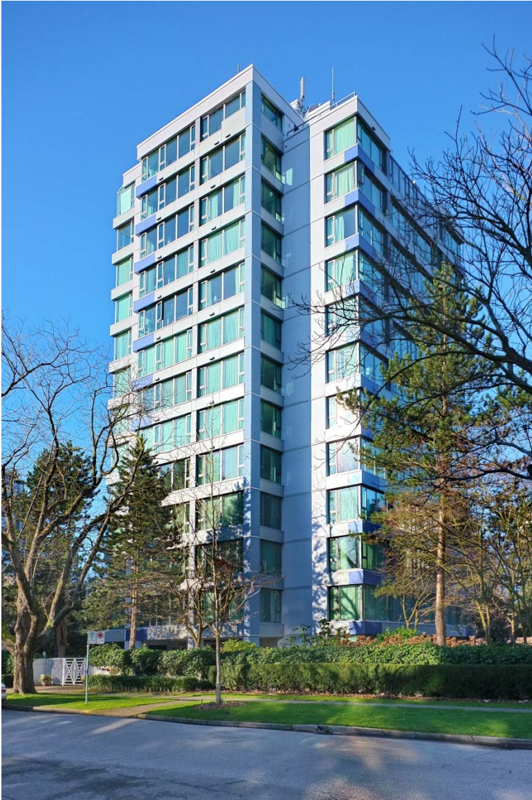
Figure 7-1: North-east corner of the case study building post-retrofit (Photo courtesy of RDH)
