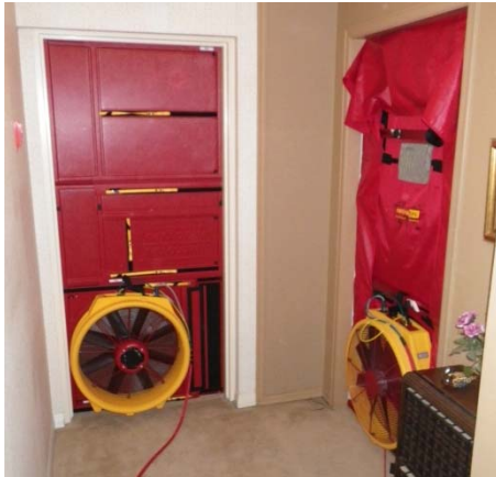
Figure 7-19: Two fan-doors used for airtightness testing of the case study building installed in a stairwell door (left) and a suite entrance door (right)
