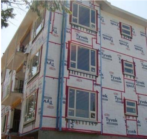
Figure 4-4: Exterior non-adhered sheathing membrane with seams taped to provide the air barrier. (Photo courtesy of RDH.)
