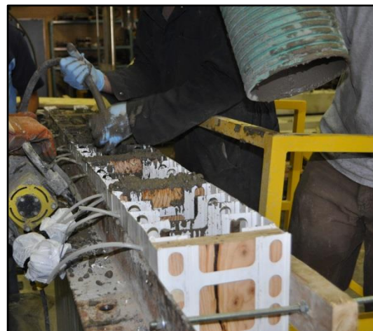
b- Vibrating the concrete
