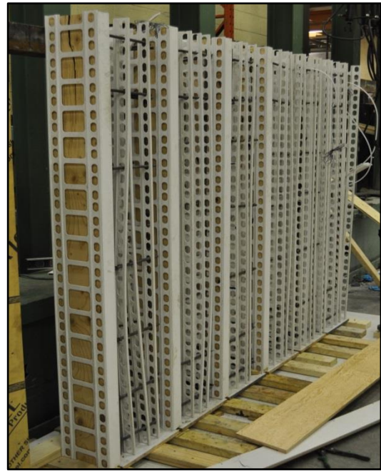
b- Assembling the PVC encased wall specimens
