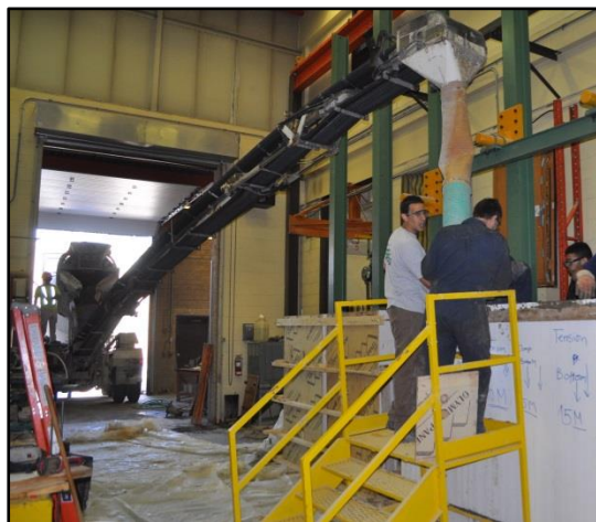
a- Casting the concrete using conveyor belt
