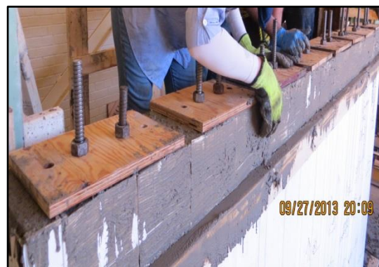
d- Placing the end plates after casting
