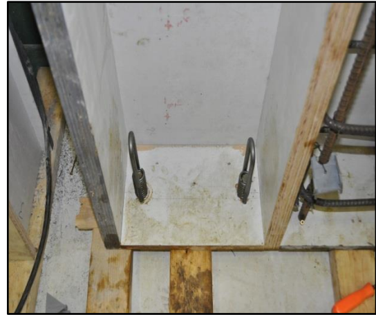
b- Base of the box with straight coil loop inserts
