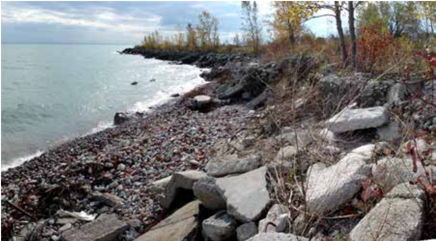
Fig. 3.7: Armoured shoreline near the causeway on the Leslie Street Spit.
