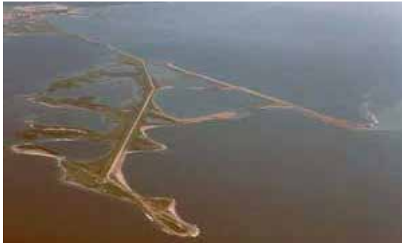
Fig. 3.4: Aerial of Leslie Street Spit while the Endikement is under construction.
