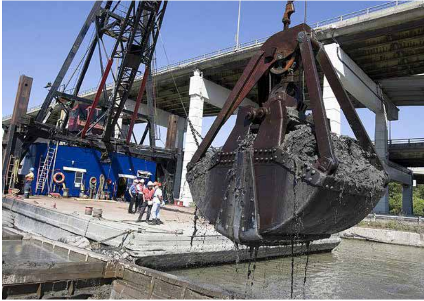
Fig. 3.26: Clamshell derrick No. 50 removing sediment from the Keating Channel.
