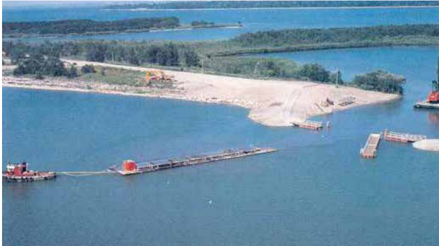
Fig. 3.28: A tugboat pulling scow barges with dredged sediment into Cell #3.
