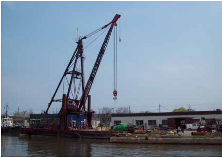
Fig. 3.25: Clamshell derrick No. 50.
