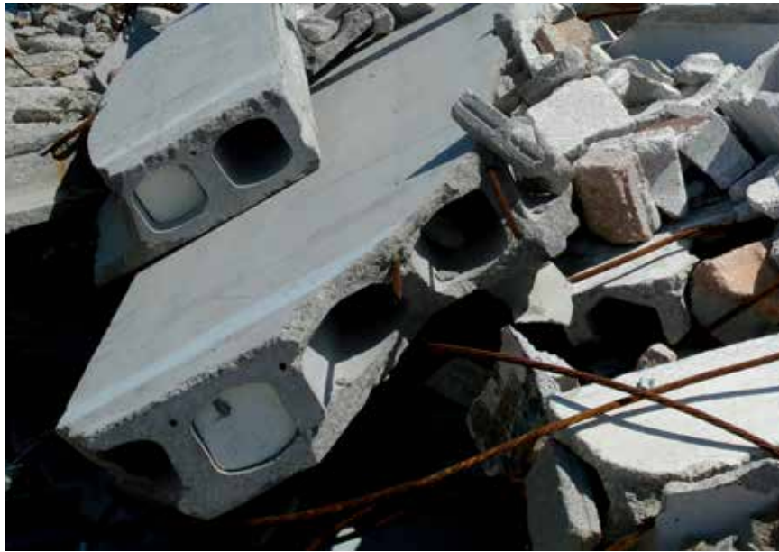
Fig. 3.12: Photo of pre-fabricated concrete slabs.
