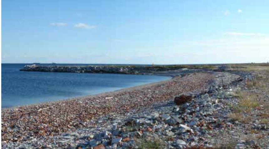
Fig. 3.9: Photo of endikement shoreline with rubble groyne visible in the distance.
