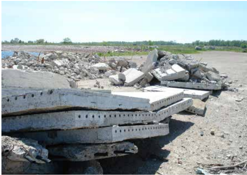
Fig. 3.11: Piles of concrete floor slabs with embedded waterheating system.
