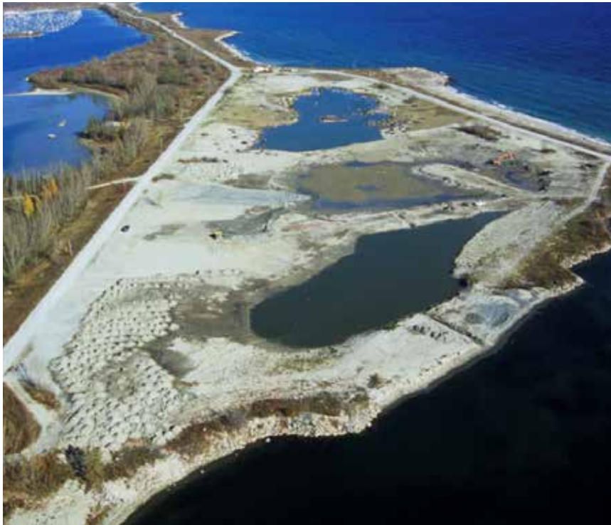
Fig. 3.44: Cell #1 in 2004 during construction.
