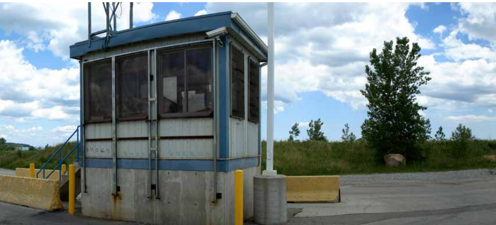
Fig. 4.16: Photo of toll gate at the beginning of the causeway.
