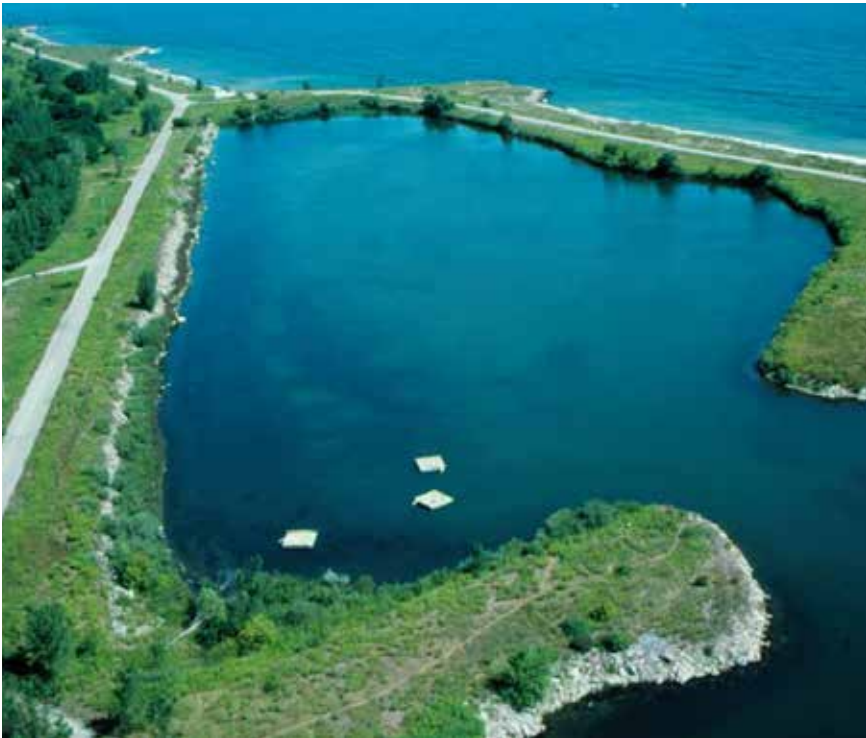
Fig. 3.43: Cell #1 in 2001 before construction.
