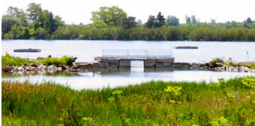
Fig. 3.47: Photo of fish and water level control structure south of Cell #1.
