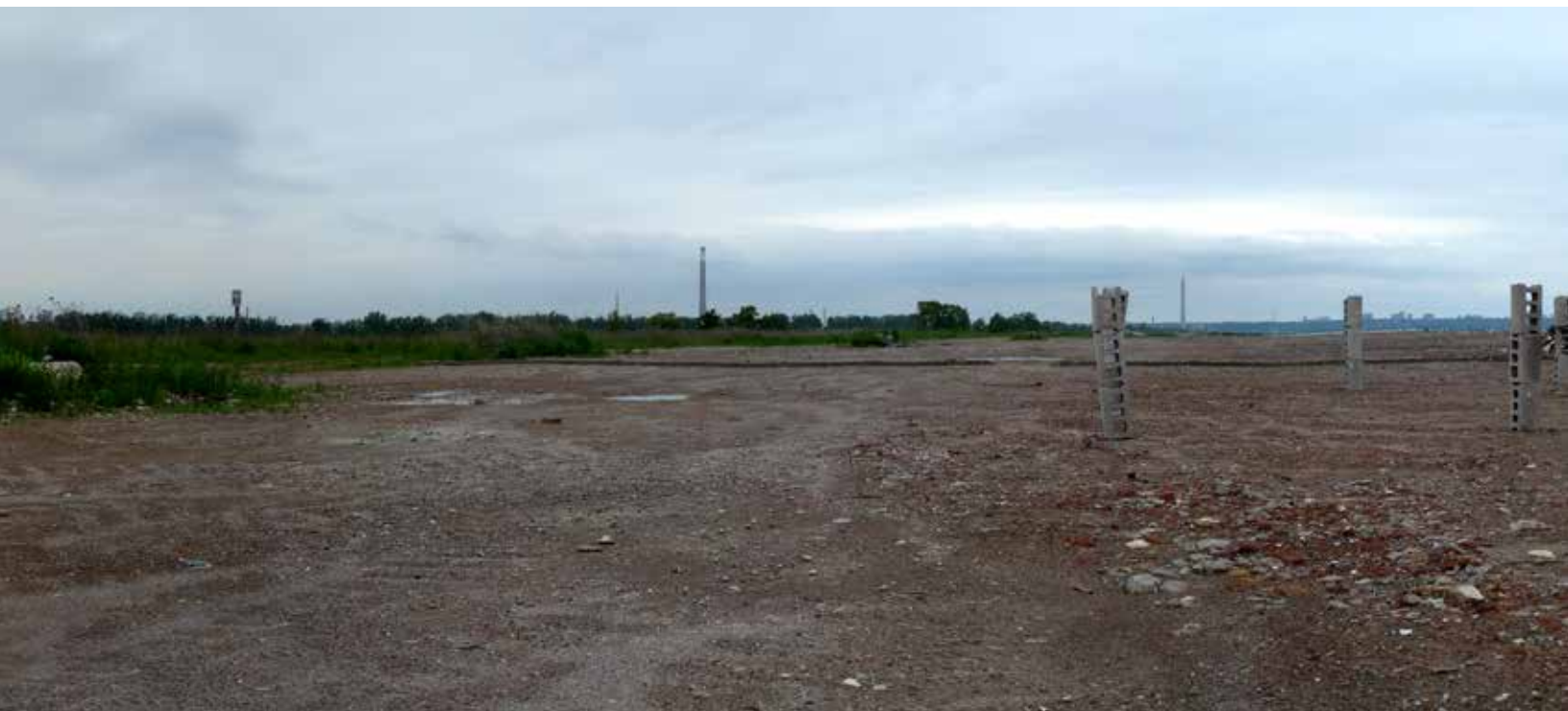
Fig. 4.22: Photo of concrete rubble on endikement.
