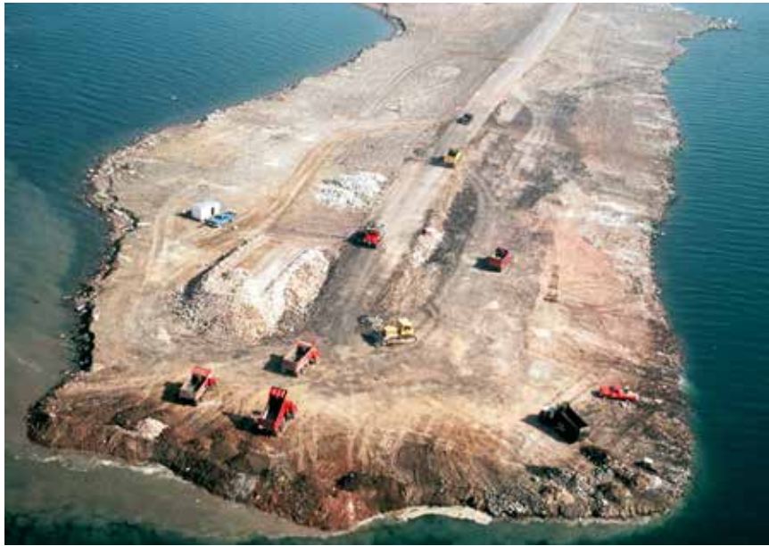
Fig. 3.2: Aerial of the southern tip of the Eastern Headland during construction.
